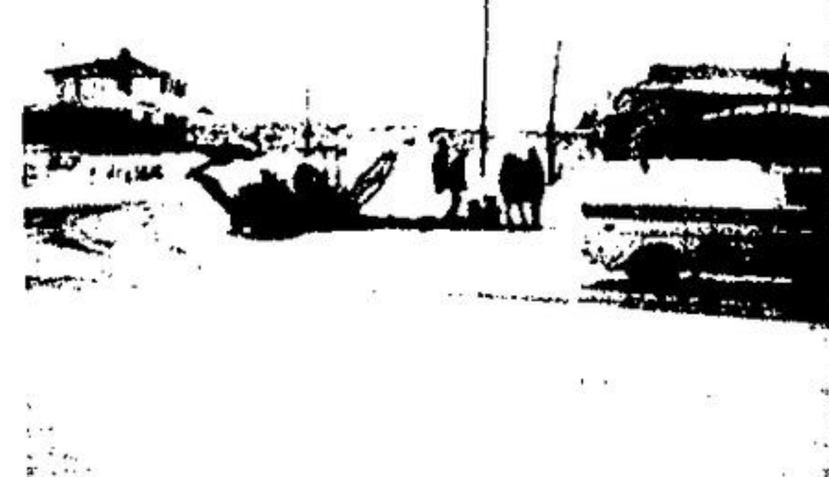
ERIC BELL COMMUNICATION has been busy installing underground cable throughout Acton. A trencher was busy in Lakeview subdivision last week.
