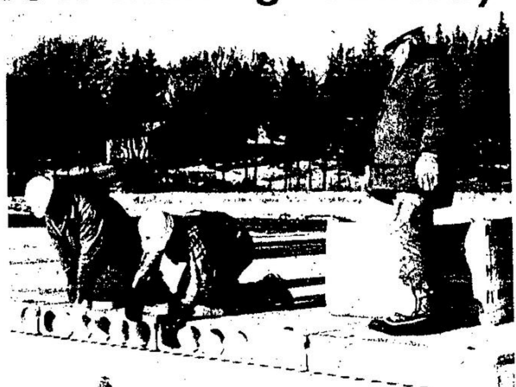
WORKERS JACK BENJAMIN, Darrell Keezub and John Charbonneau of Toronto place styrofoam plugs in the ends of the cored rods of the floor slabs on Monday at the Lions Club community centre. Next step will be to pour two inches of concrete over the floor and, if weather permits, the Lions will proceed with side walls.
