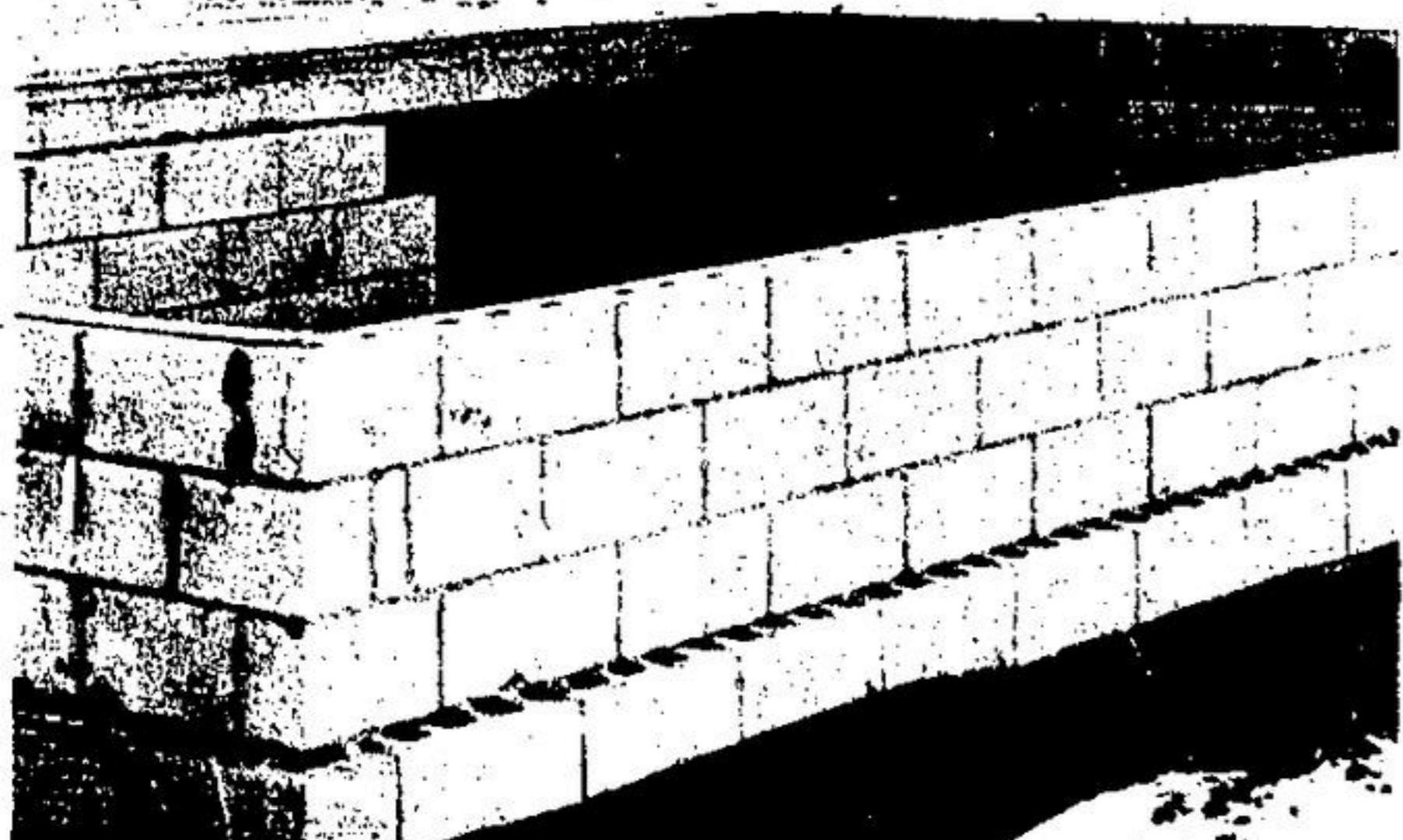
SLABS WEIGHING one ton apiece were delivered and placed as the first-floor foundation of the Lions Club community centre last Monday. It took a 150-foot crane to pick up the immense tailor-made slabs and set them in their proper place. Each piece was notched for vertical posts and reinforced with steel rods cored out for purposes of sound-proofing.
