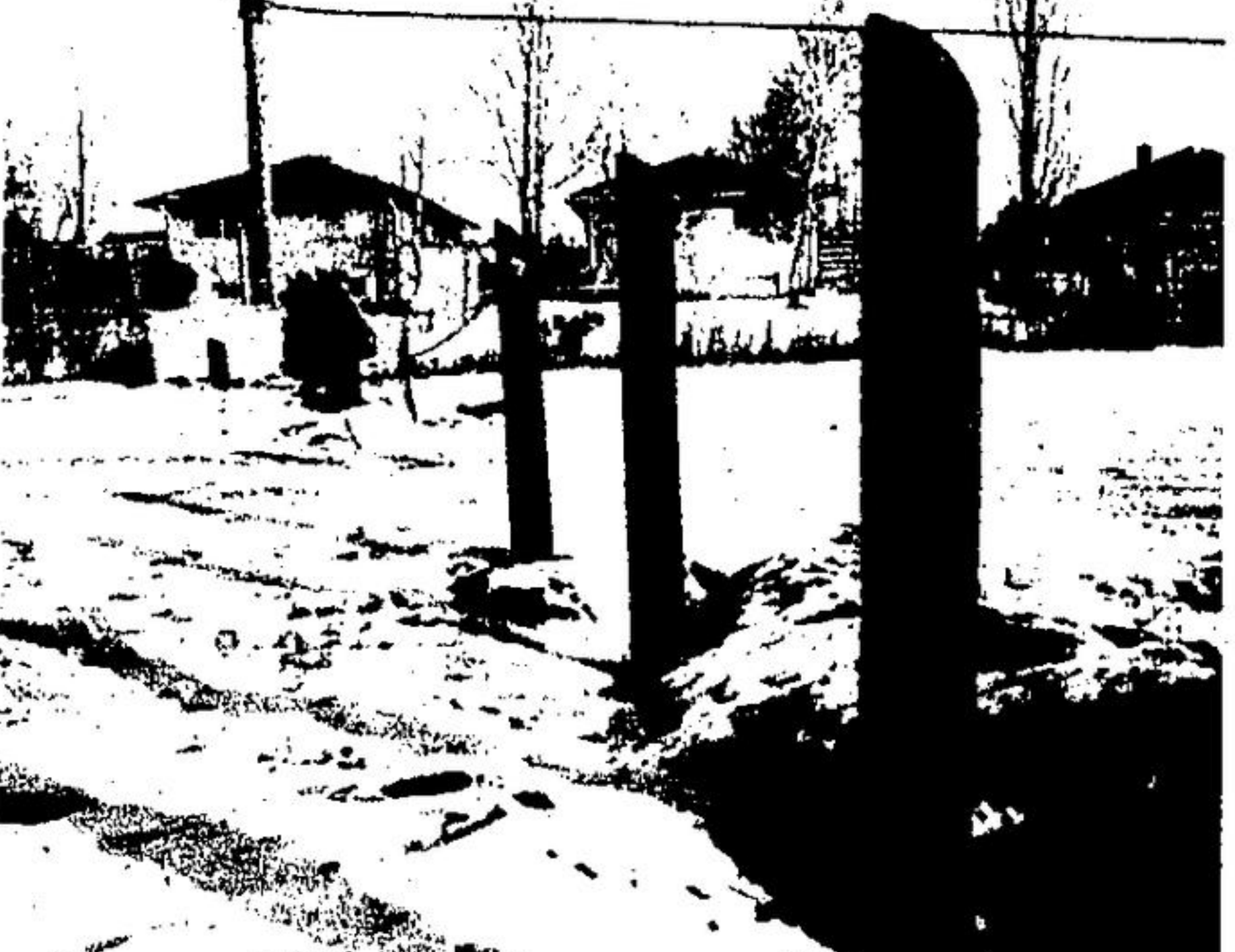
NEW CEDAR post and chain link fence has been erected at the entrance to Sir Donald Mann park in Glenlea subdivision. Its purpose is to prevent trucks entering the park and playground area. Recreation director Doug Collison expects there'll be vandalism of the fence.
