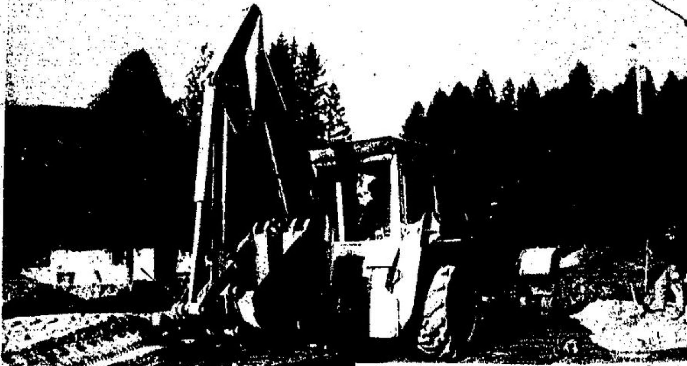
CORNER OF MILL W. and Cobblehill Rd. is getting a facelift as its part of the road improvement program, currently underway. New ditches and culverts will make the road ready for heavier traffic, due to Kingham Hills subdivision.
