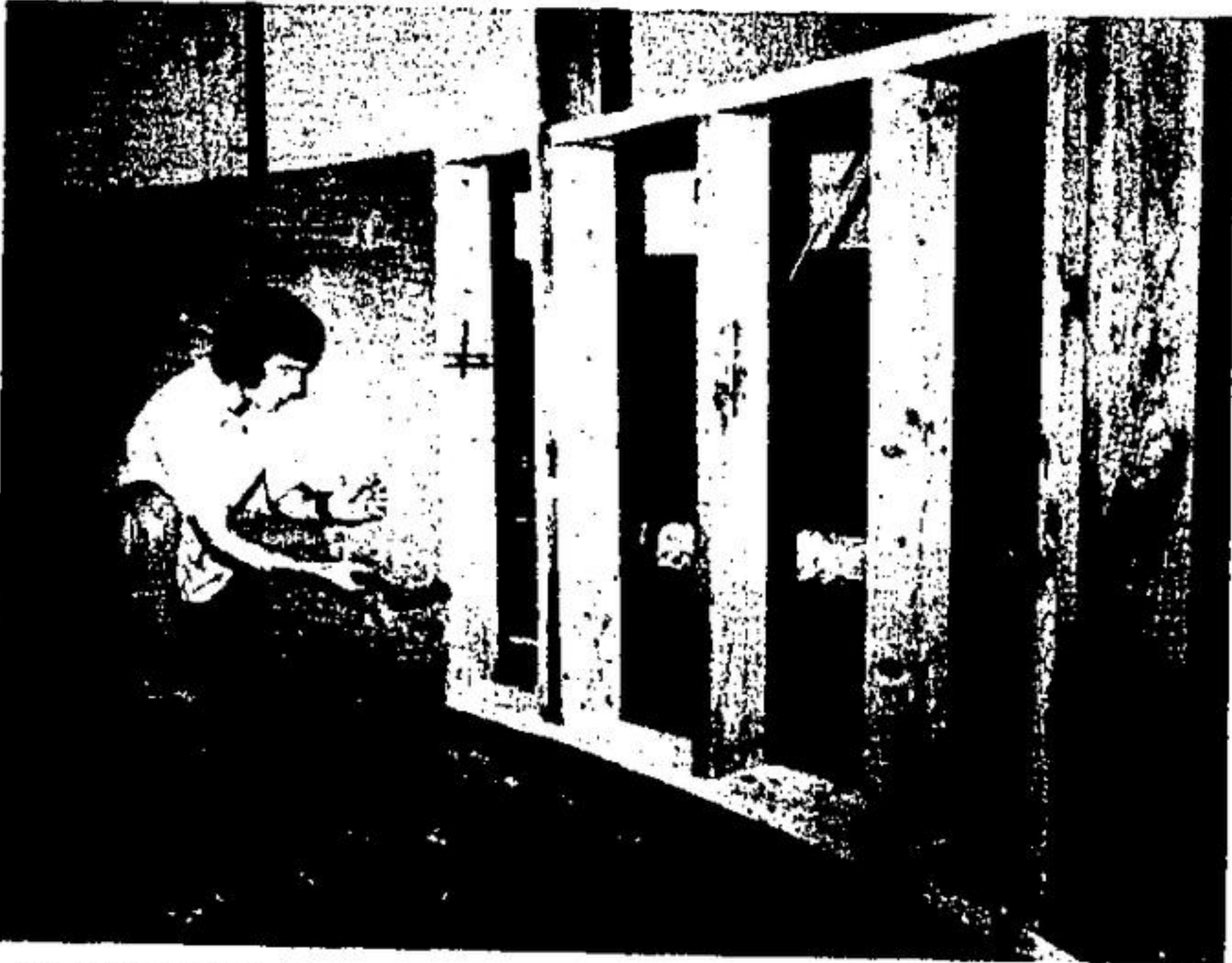
NEW BOARDS SHOULD all be installed in the arena by today, and ice making equipment will be turned on right away. If the weather stays cold, there could be a sheet of ice by next Tuesday. Kevin Lumbers is the contractor making the changes in the arena. Plastic boards are expected to be better than the previous wooden ones.
