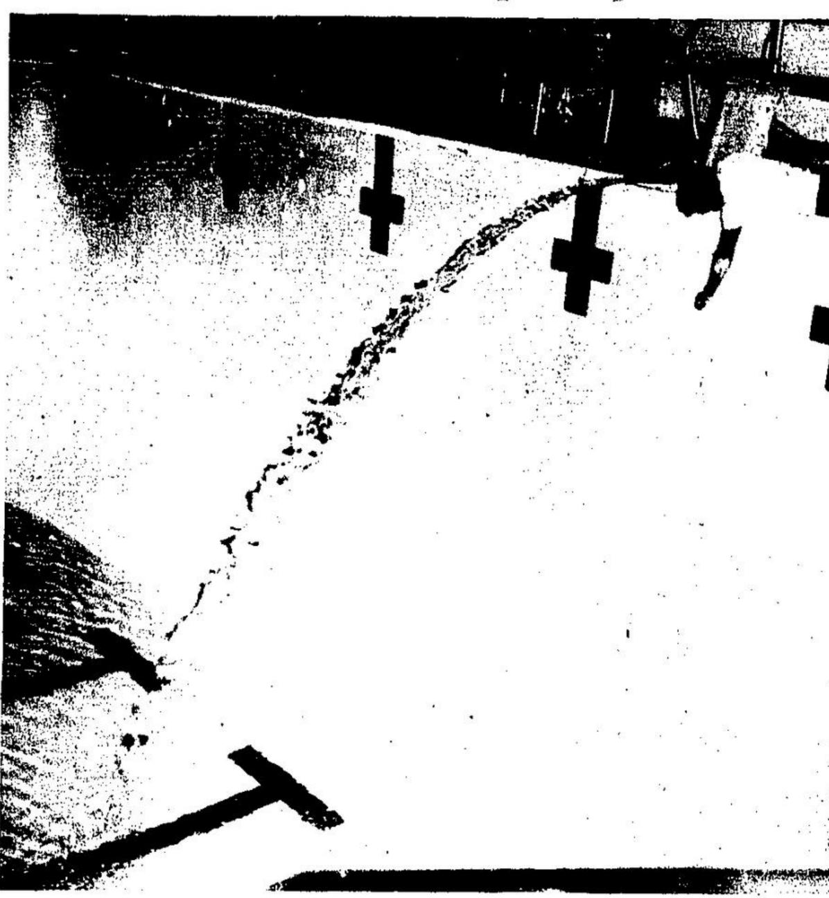
FIRST WATER POURED INTO the Lions centennial pool Thursday afternoon immediately after the pool had been lined. The cool water cures the marmorite lining. The pool has a 170,000 gallon capacity with a 13 foot depth at one end, graduating to three feet, six inches at the
