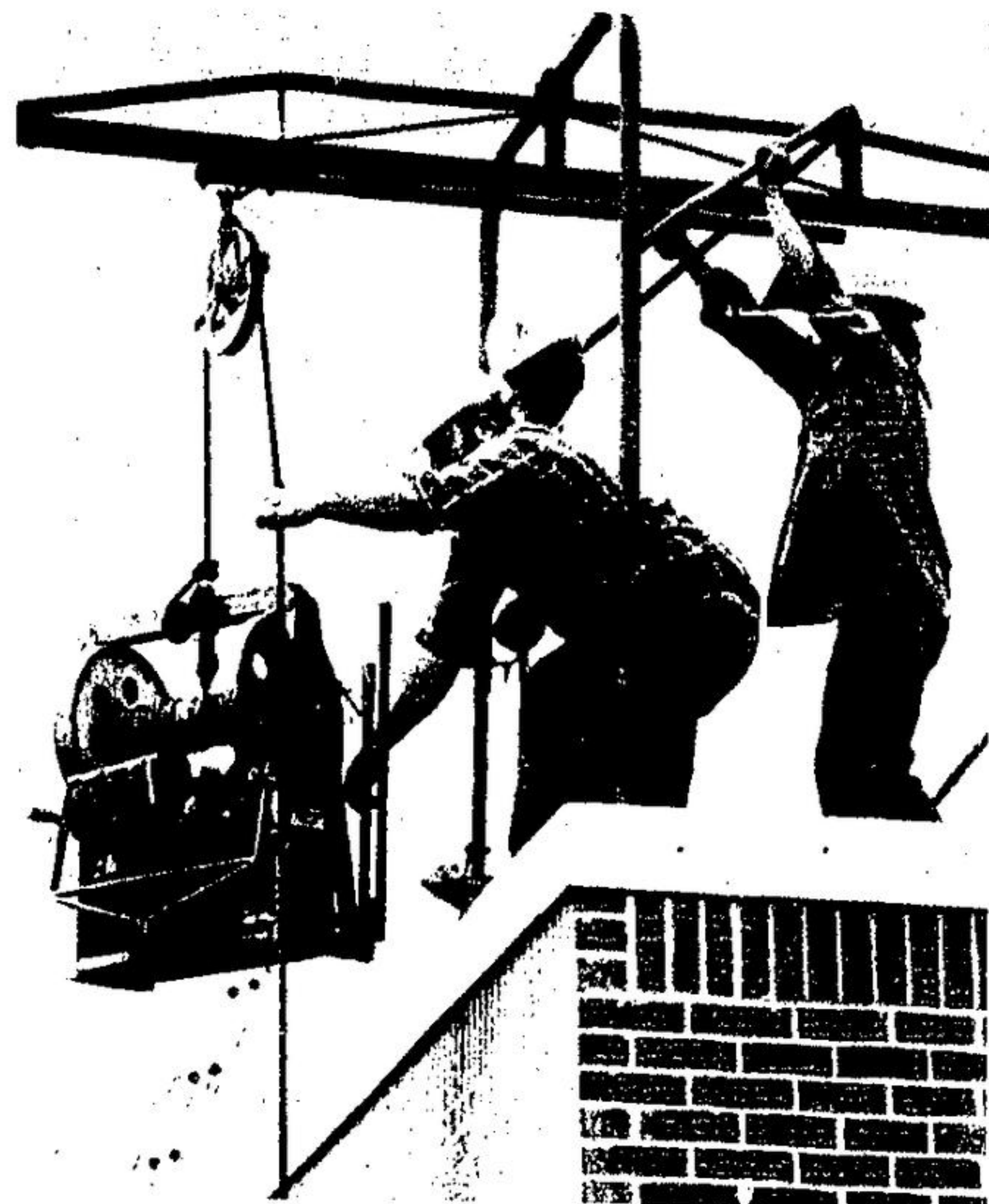
WORKMEN ARE pictured last week preparing to tar the shower and change room rooves at the new swimming pool. Problems have plagued progress but work continues.
