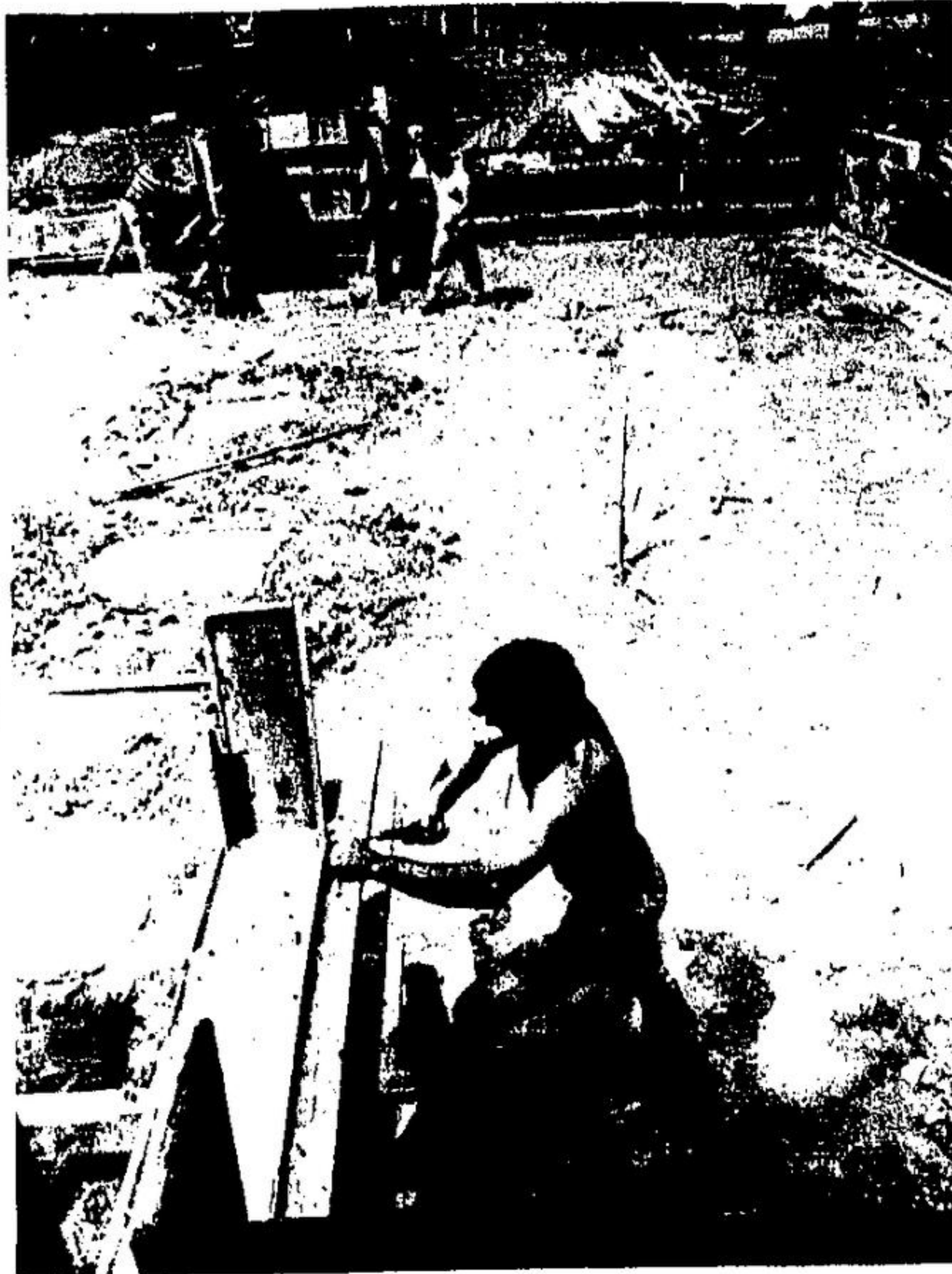
NEW MEDICAL centre on Mill St. is taking shape, with Pawlowski Construction of Kitchener the contractors. Tom Parker removes frames from footings and basement walls. Acton Medical group will move here from their cramped quarters at Mill and Main corner.
