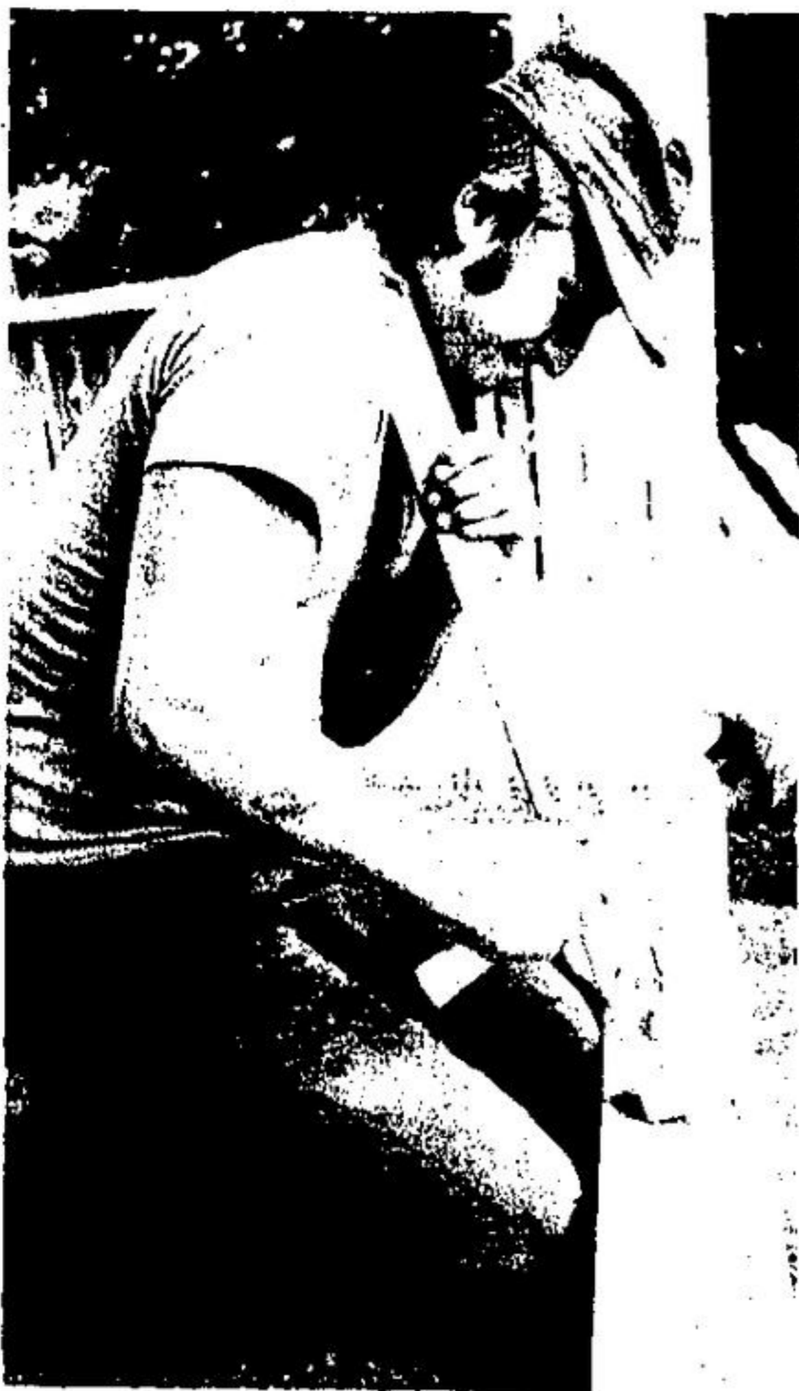
DANNY HILLIER has that concentrated look of a man trying to hammer in two by two's successfully. This is part of the new railing on the top of the bandshell.
