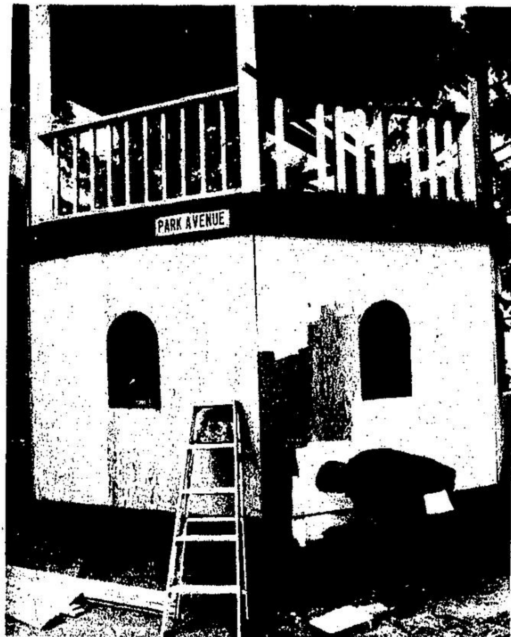
TOWN EMPLOYEE Sam Tennant is hard at work putting on the flat coat for the bandshell. The effort will be well worth the result. Halton Hills Works Committee ordered the facelift for the bandshell at the park gates.
