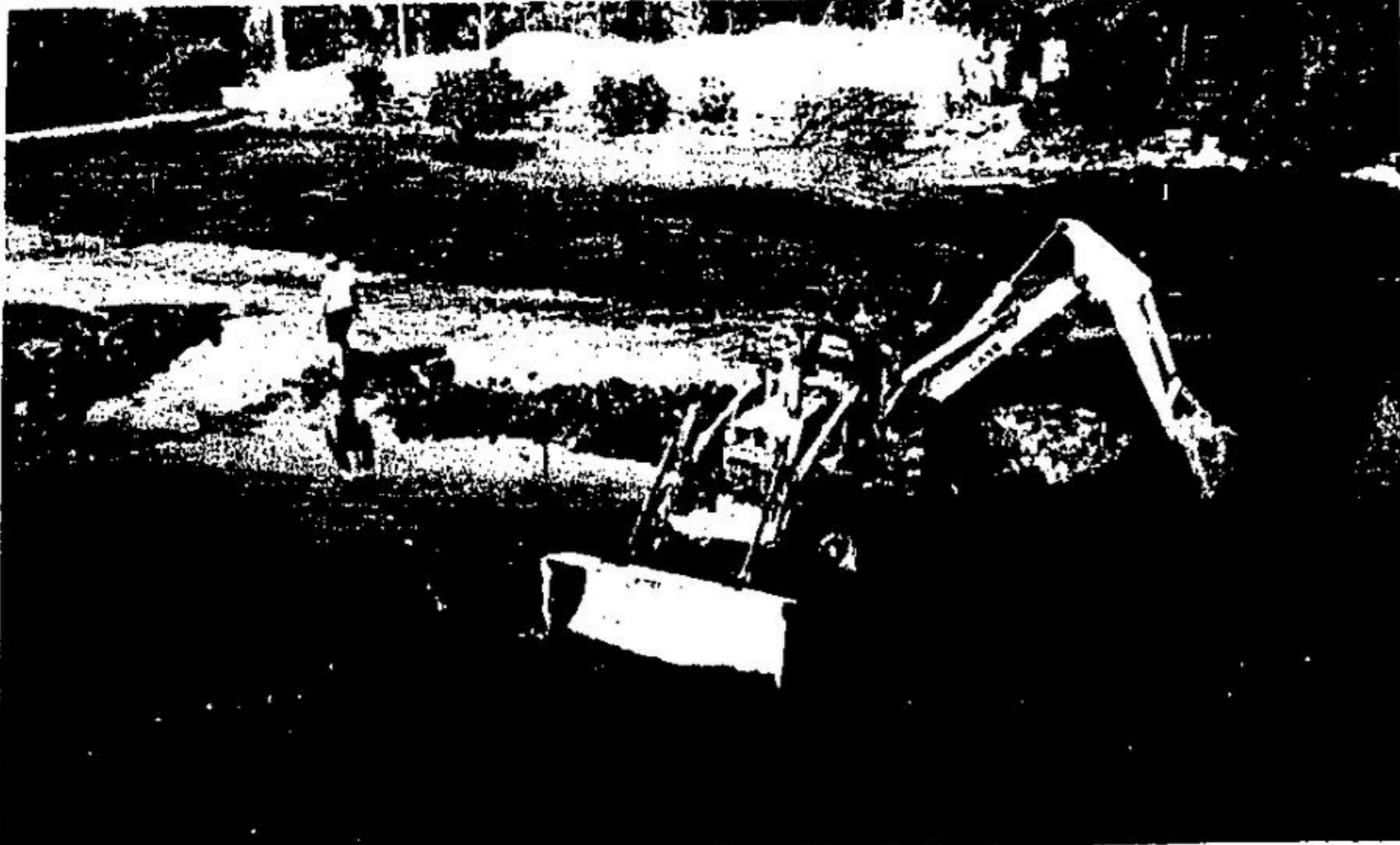
REMOVAL OF A piece of wood caught in the water wheel of the James Milne and Son mill on Main St., required draining the water bed and digging with a bulldozer Tuesday. Besides wood re-
