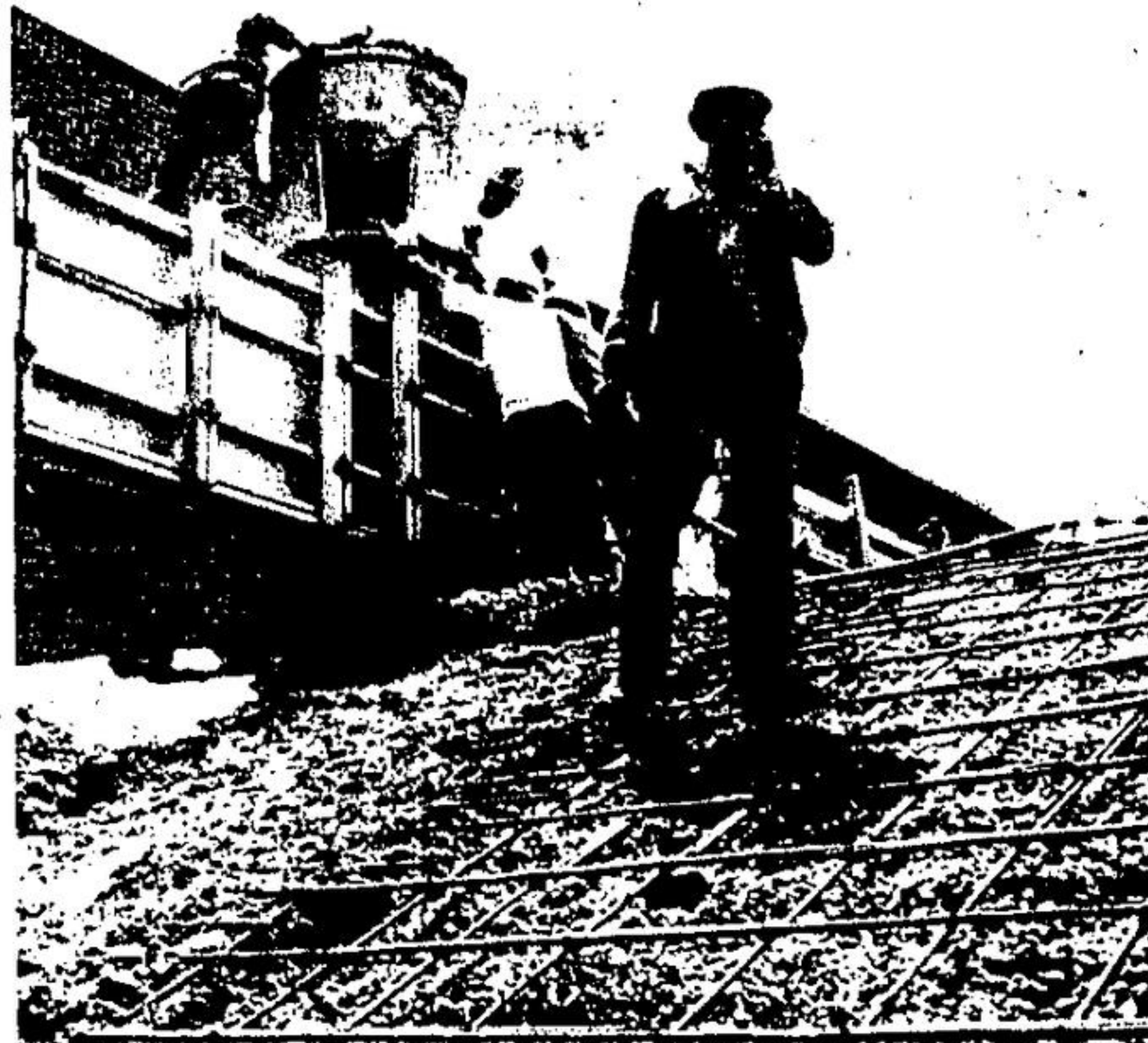
SLOPING GRADE for the Lions centennial swimming pool was poured by workmen last week. The pool, adjoining the high school, is the Lions project for the town's centennial.
