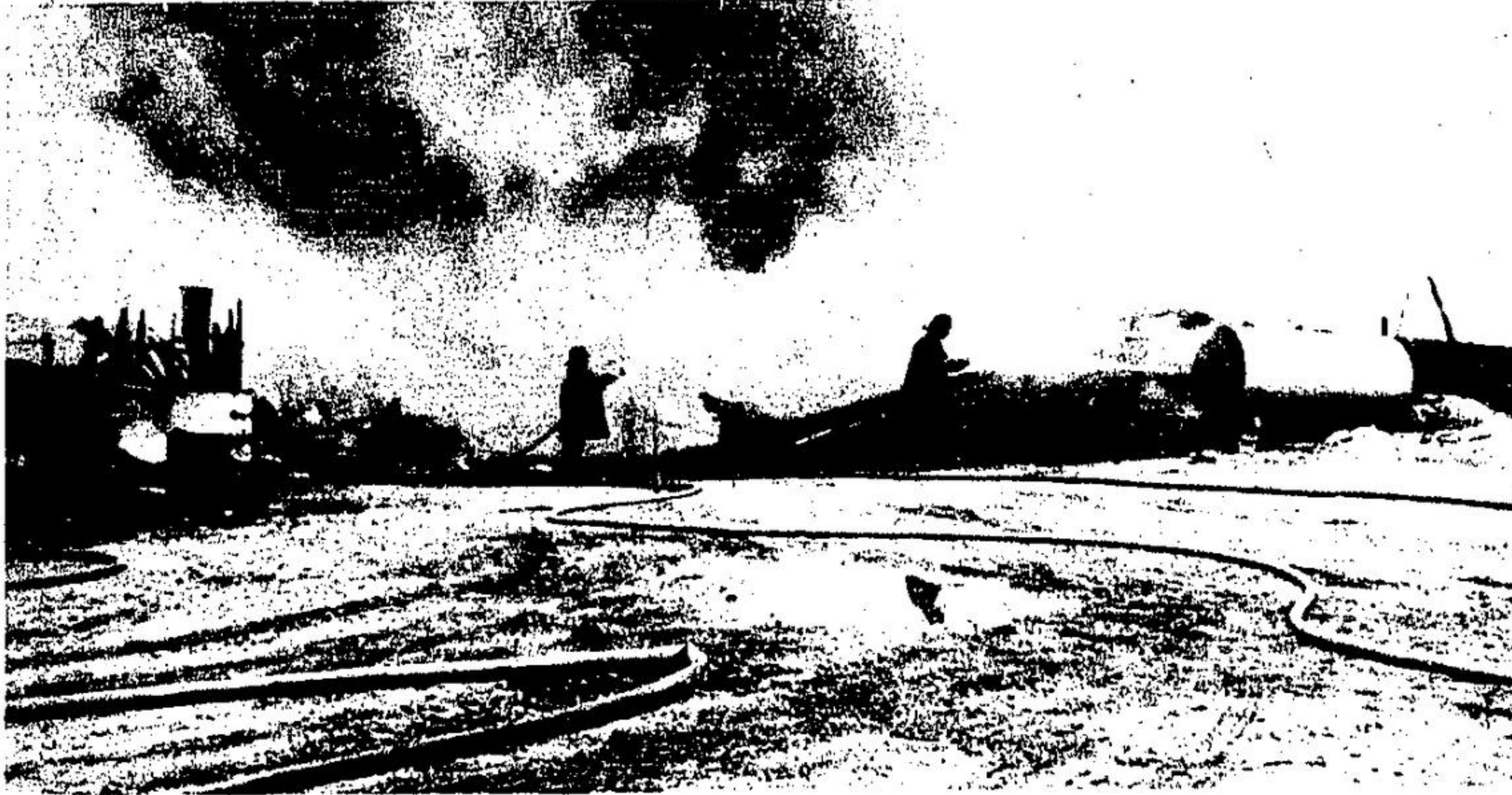
FIREFIGHTERS spray the charred remains of a Nassagaweya pig barn and implement shed Friday afternoon. Damage to the property of H. C. Smith, Second Line, is estimated at about $50,000. Milton and Acton firefighters were unable to save 578 hogs in the barn and a number of pieces of farm machinery. None was at home when the blaze started.
