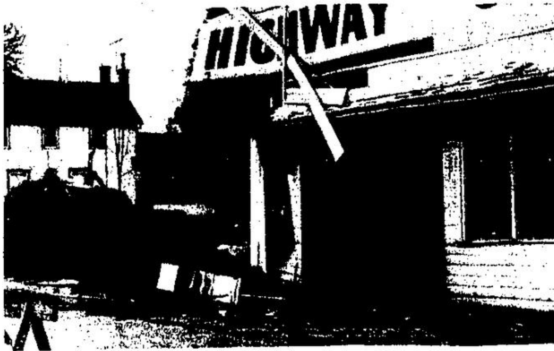
HIGHWAY GARAGE is no more. This site has been taken over by Alteo Construction, owned by Alf Berry. Mr. Berry plans work to start immediately on an office building for his company.
