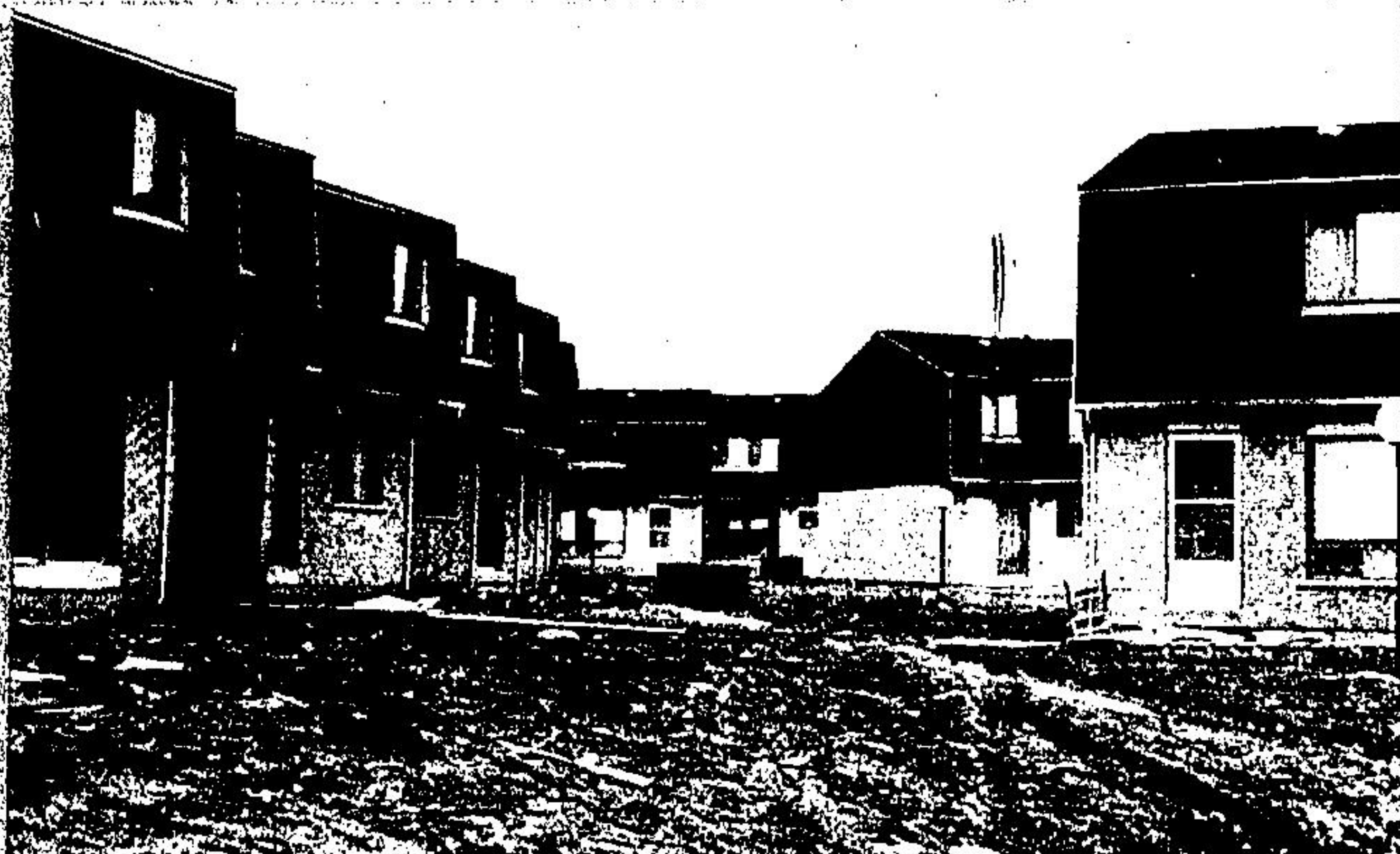
Town houses nearing completion off Mountainview Dr., Georgetown.
