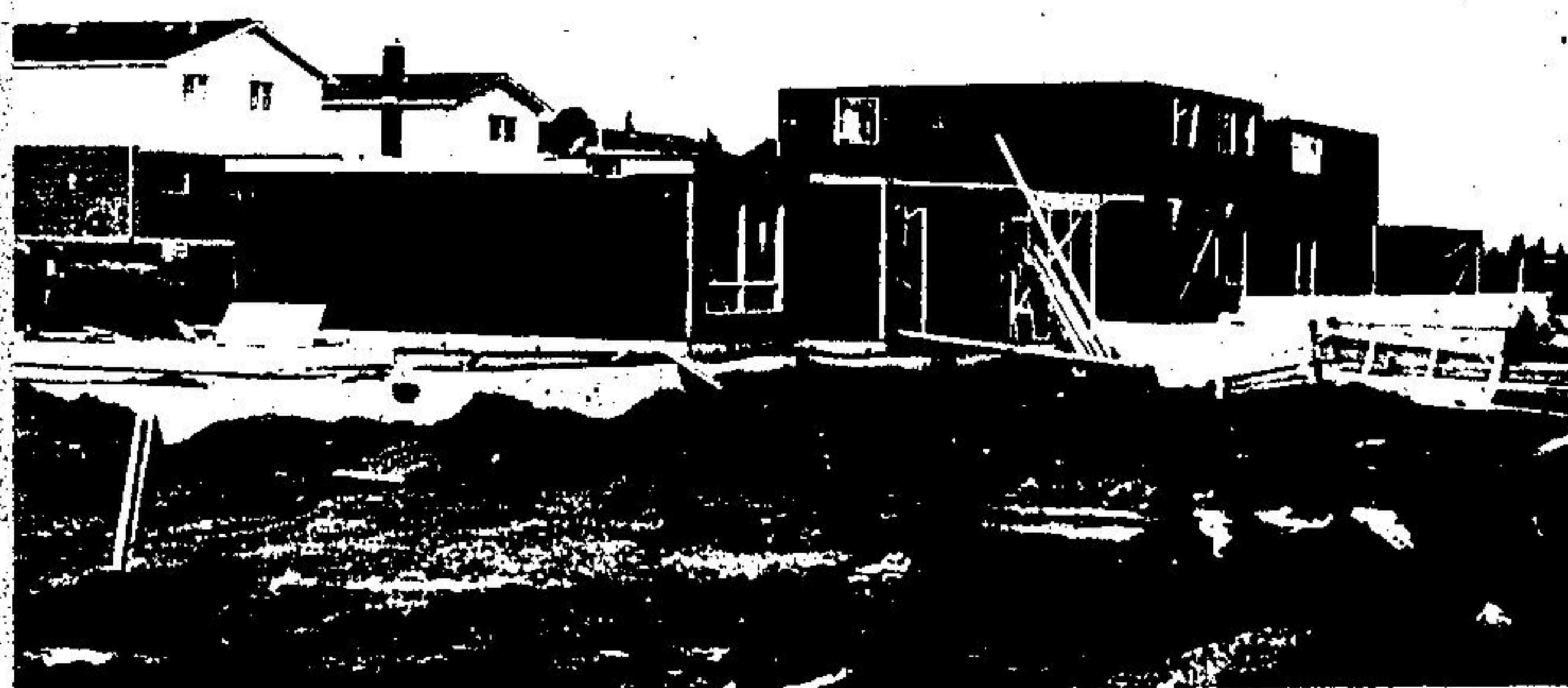
Single family houses are rising on Cobble Hill in Acton.
