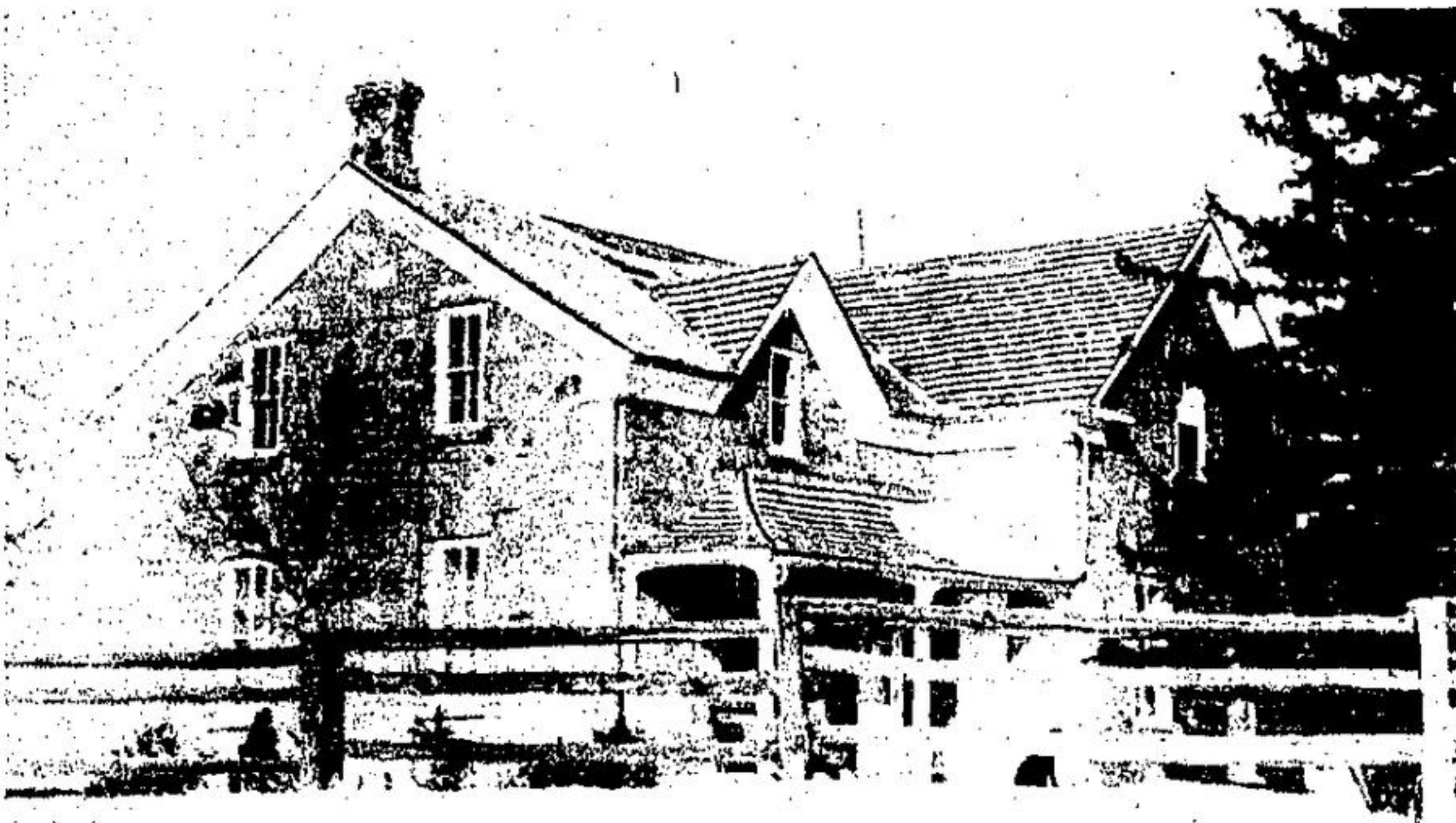
CEDAR CREEK FARMHOUSE on Fourth Line, Esqueving Township was built in 1870 by James Warren. He emigrated to Canada in 1832 and lived in a log house un-
