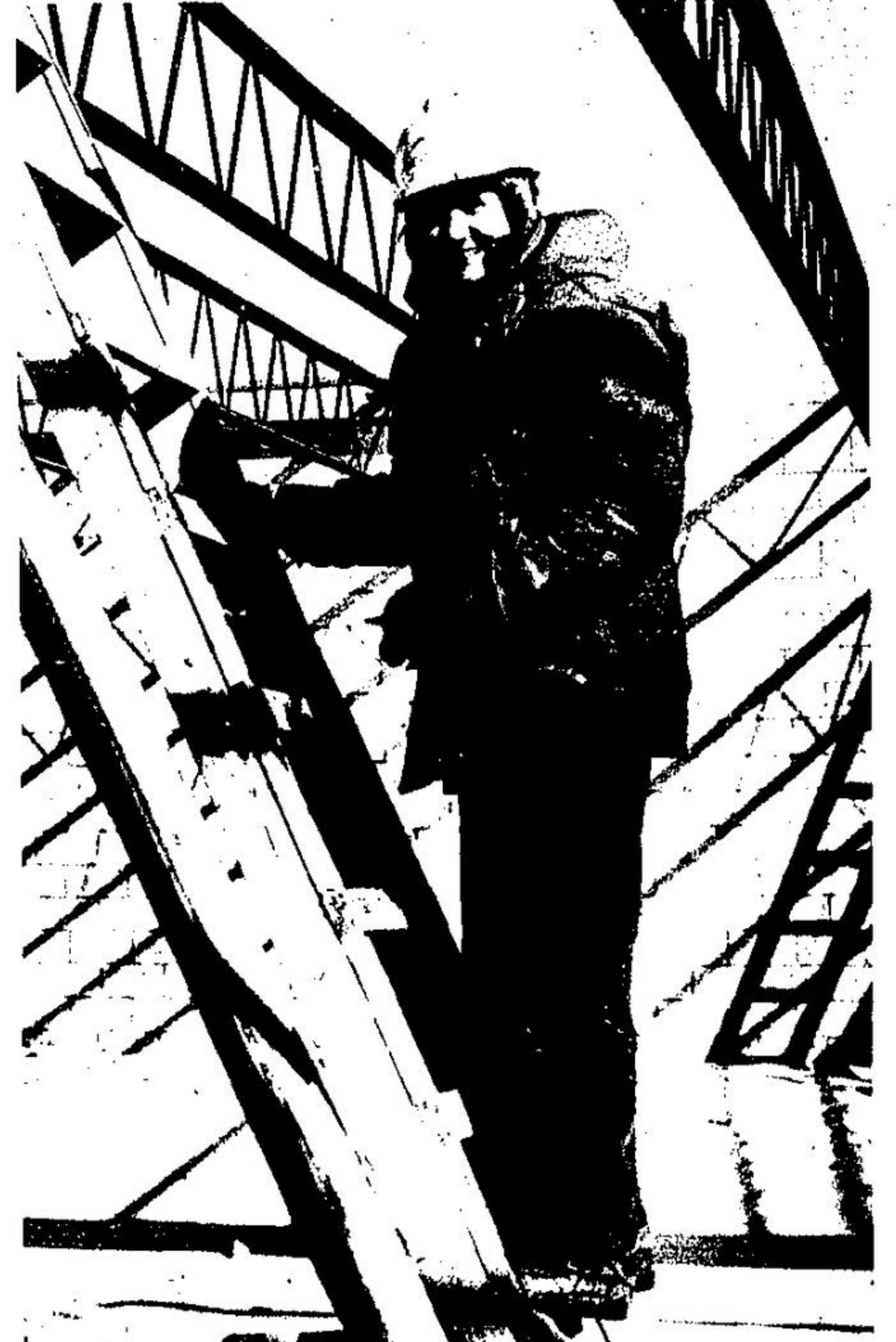
PRETTIEST steel installer around, Heike Bollert has been working with her father Gus who has the contract for the steel framework at the new Legion hall. Soft-spoken Heike graduated from grade 12 and decided she'd like nothing better right now than to work outdoors with her dad. Right, she is bundled up against the weekend zero weather as work continues. Left she's silhouetted against the frosty sky. Heike turns 19 this Friday.
