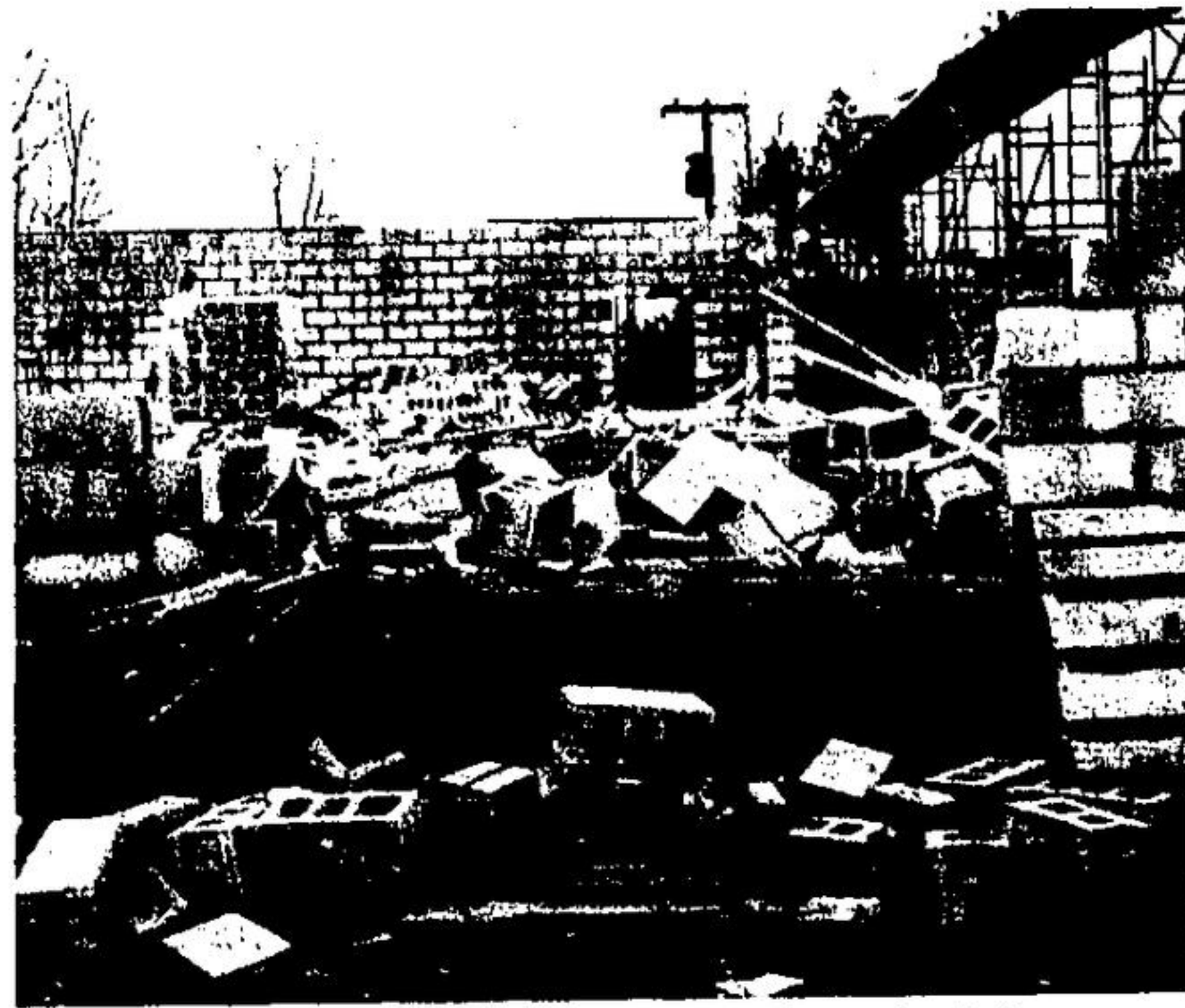
INTERIOR wall of Limehouse school collapses in wind.
