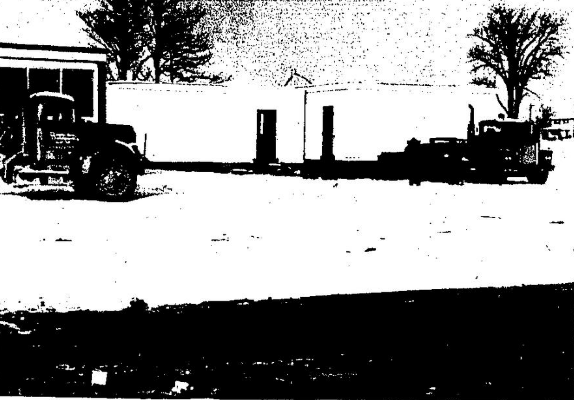
LOCATION OF THE new swimming pool behind the high school is bared, as the two portable classrooms were moved Monday to a new location a few yards further north. Bare ground in front reveals the site of the Lions centennial swimming pool project. A canvass will begin this winter.
