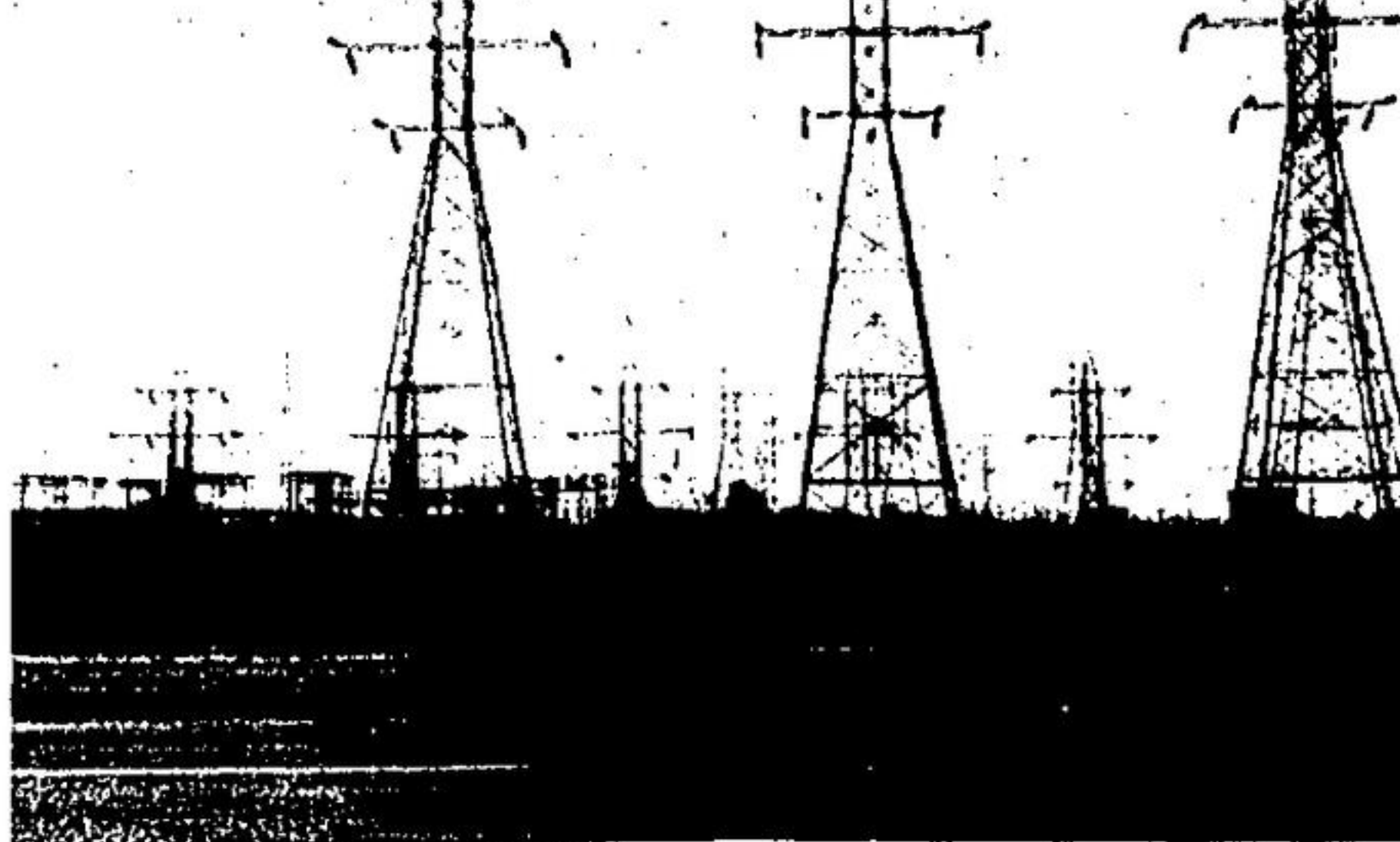
These Hydro sentinels march through Burlington.
