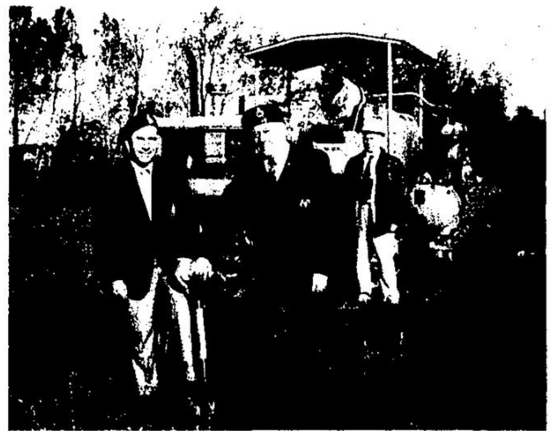
THE DIE IS CAST. Tuesday morning president Bob Angell and Mayor Les Doby turned the first sod to get the new Acton legion hall off the ground on the 10 acre site, west of Cameron Avenue, beside Fairy Lake and opposite Prospect Park. Operating the bulldozer in the background is Lloyd Nellis and, beside the machine is Percy Jinks, official superintendent of legion hall building. He recently completed another hall in Agincourt. Percy will be in charge of the local project for the Legion Branch No. 197 here in Acton. (Photo by L. Root)
