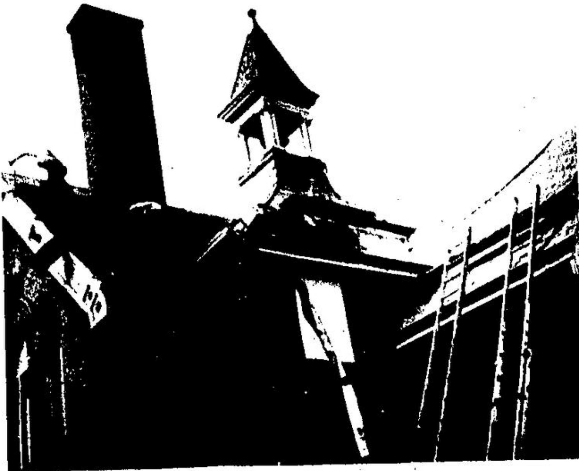
THE SLATE ROOF which has covered Knox Presbyterian Church since it was built in 1894 is being ripped off this week and replaced with new self-sealing asphalt shingles. The slate was becoming badly cracked and creating leaks. Nick Owens and Tom Browning of Western Contracting are the roofers shingling the 7,600 square foot roof. The slate roof was one of the few remaining in the Acton area. —(D. Gibbons Photo)
