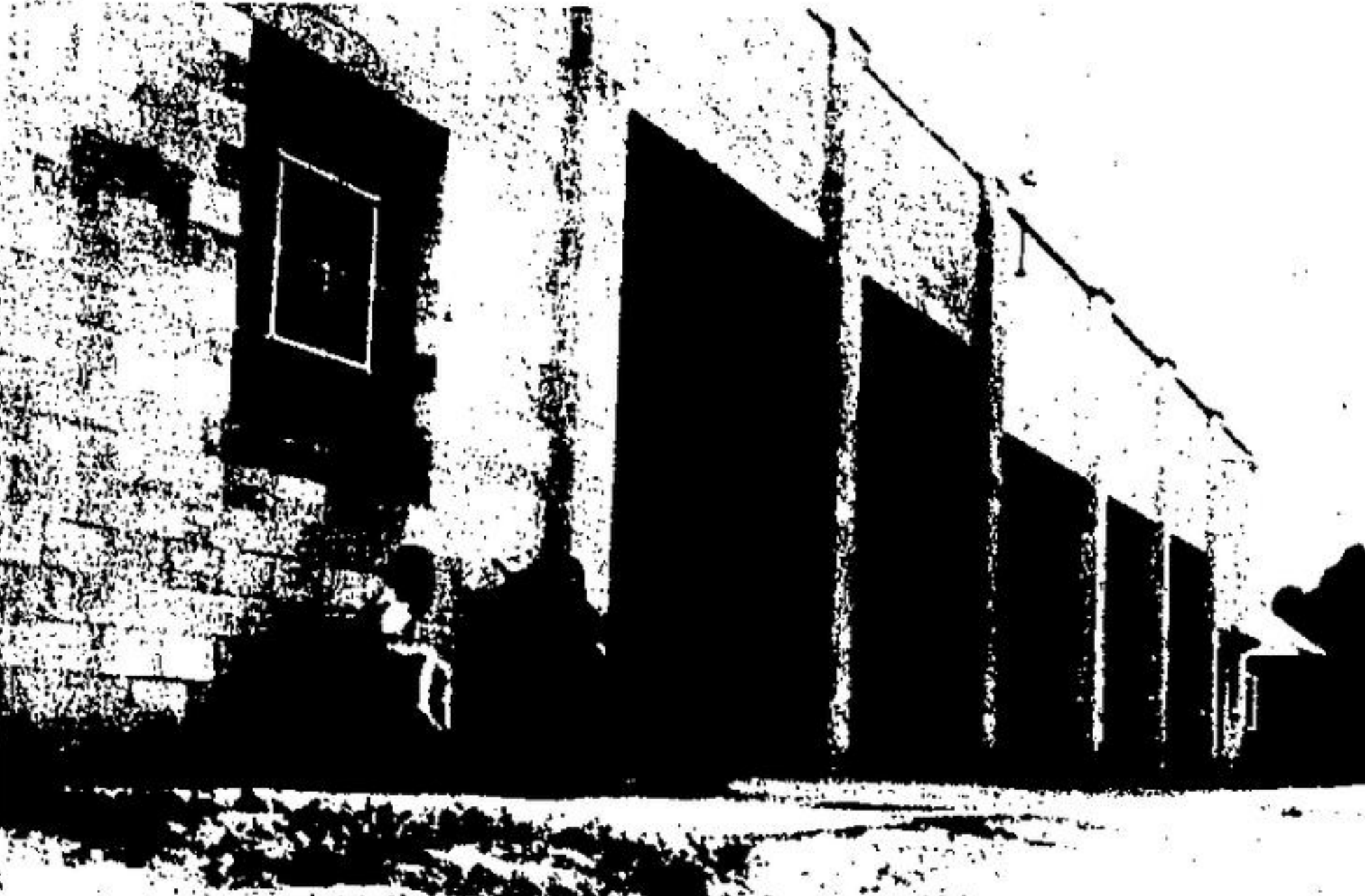
A RECENT EXPANSION took place at Nassagaweya Township roads department's garage and headquarters building at Brookville, and this Saturday afternoon an open house is planned by the staff and councillors. In the evening a
