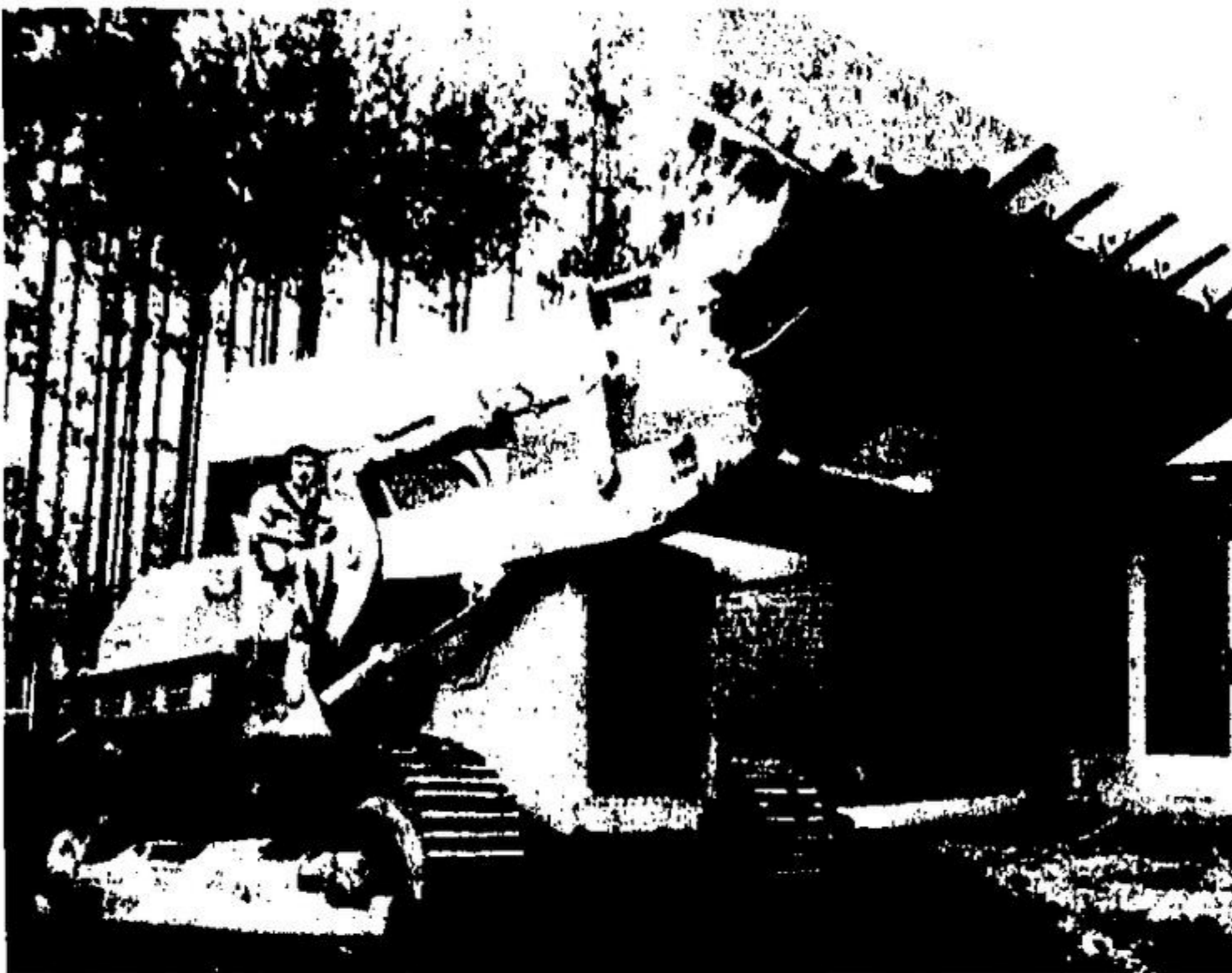
DOWN, UP, AND INTO THE TRUCK, and already the ground is almost dug to completion for the base of the four room addition to the Rockwood Centennial School which should be completed by August 15.
