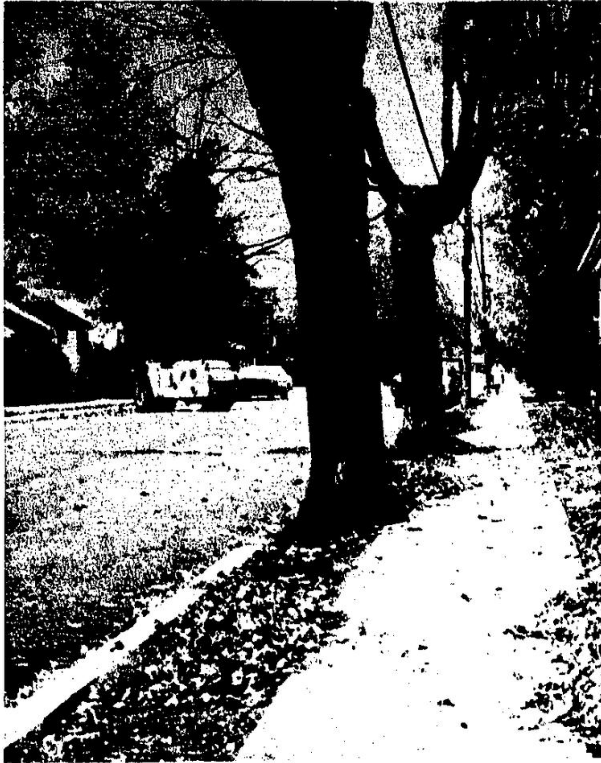
WORKMEN PUT THE FINISHING touches on Bower Avenue paving this week as the $68,544.20 job on street reconstruction is in its final stages. New sidewalks and curbs, underground wiring and a wider road have all combined to make it one of the finest streets in town. Many of the fine old maples on the Bower were preserved despite the face lifting. (Photo by J. Jennings)
