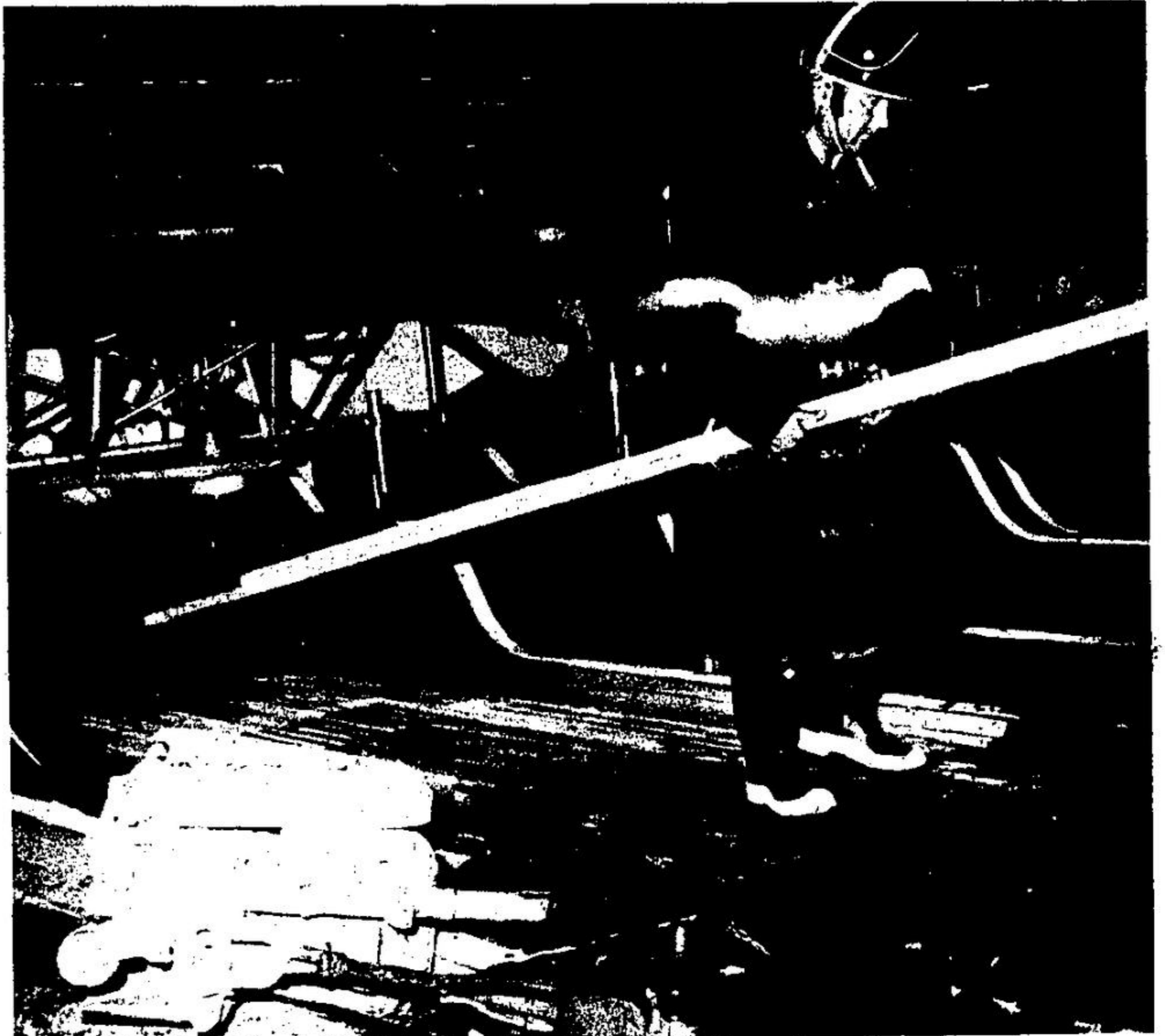
ACTON BOWLING Lanes received an estimated $10,000 damage Friday afternoon when a sanding machine operated by 32 year old Denis Maurice of Toronto exploded. Mr. Maurice received third degree burns to 80 per cent of his body. He died in Hamilton General Hospital Sunday, Checking damage to the building and the machine (foreground) is by firefighter John Krapek. (Photo by D. Pink)
