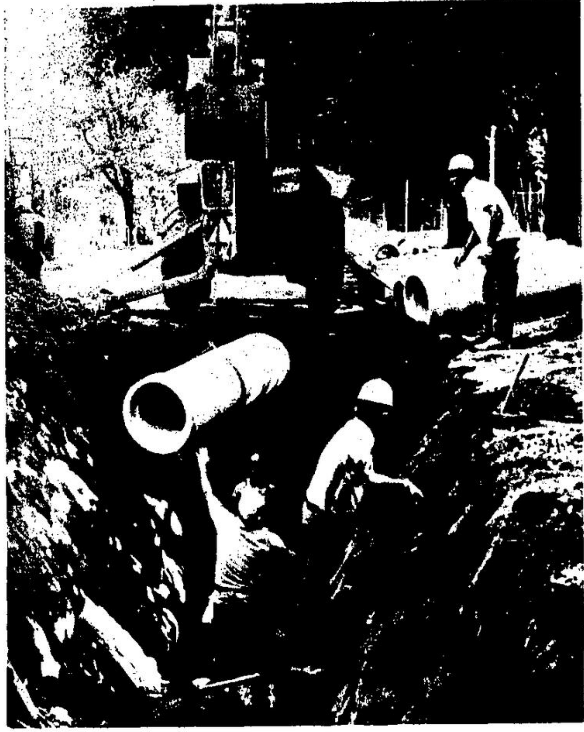
WORKMEN are laying storm sewer pipe along Church St. to accommodate the new apartments. A large area of the street has been blocked off while work is in progress. (D. Pink Photo)
