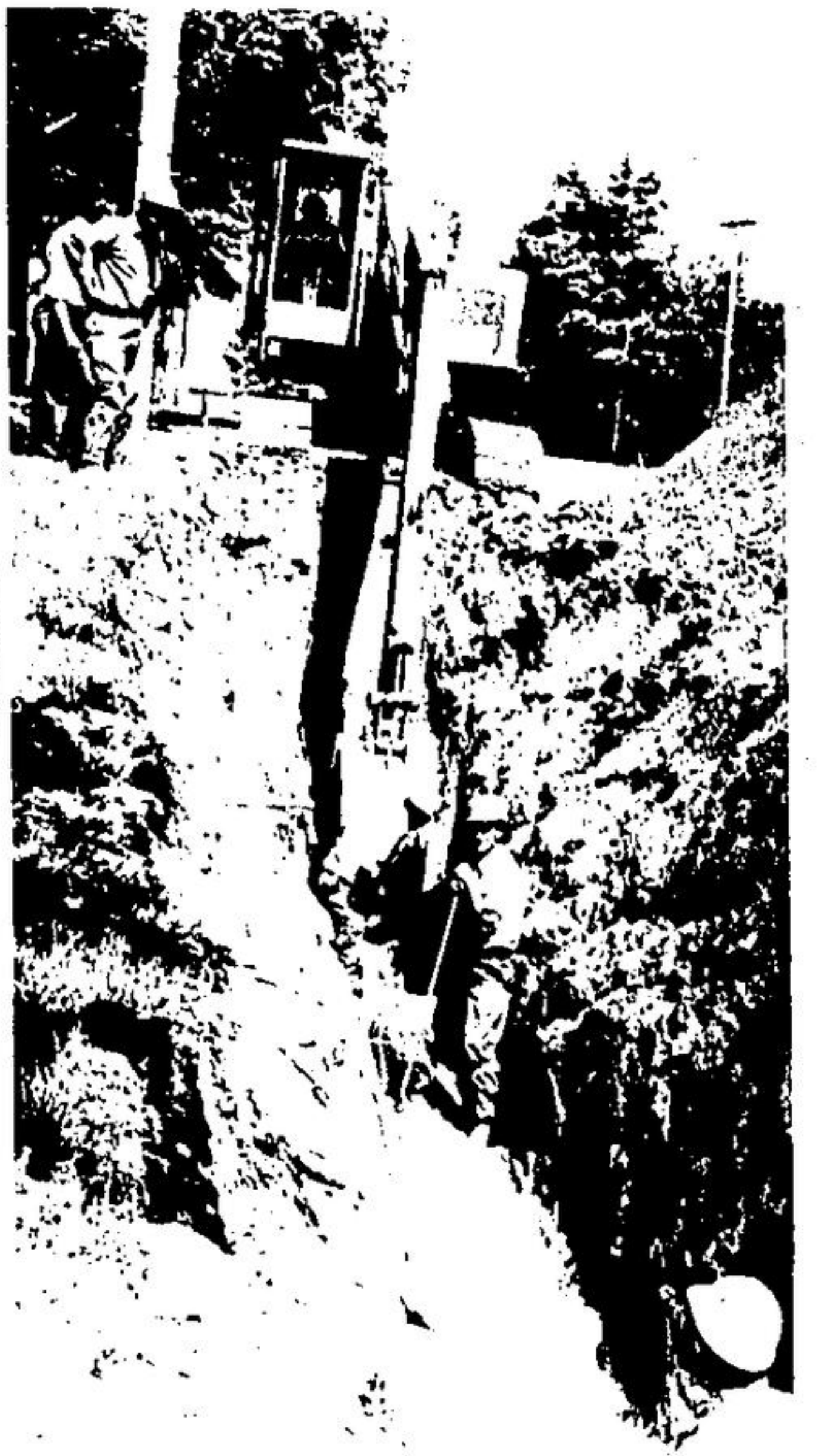
TWINBEE Construction workers began laying the new water line which will connect the town reservoir with a new well on the Fourth Line of Erin township last week.
