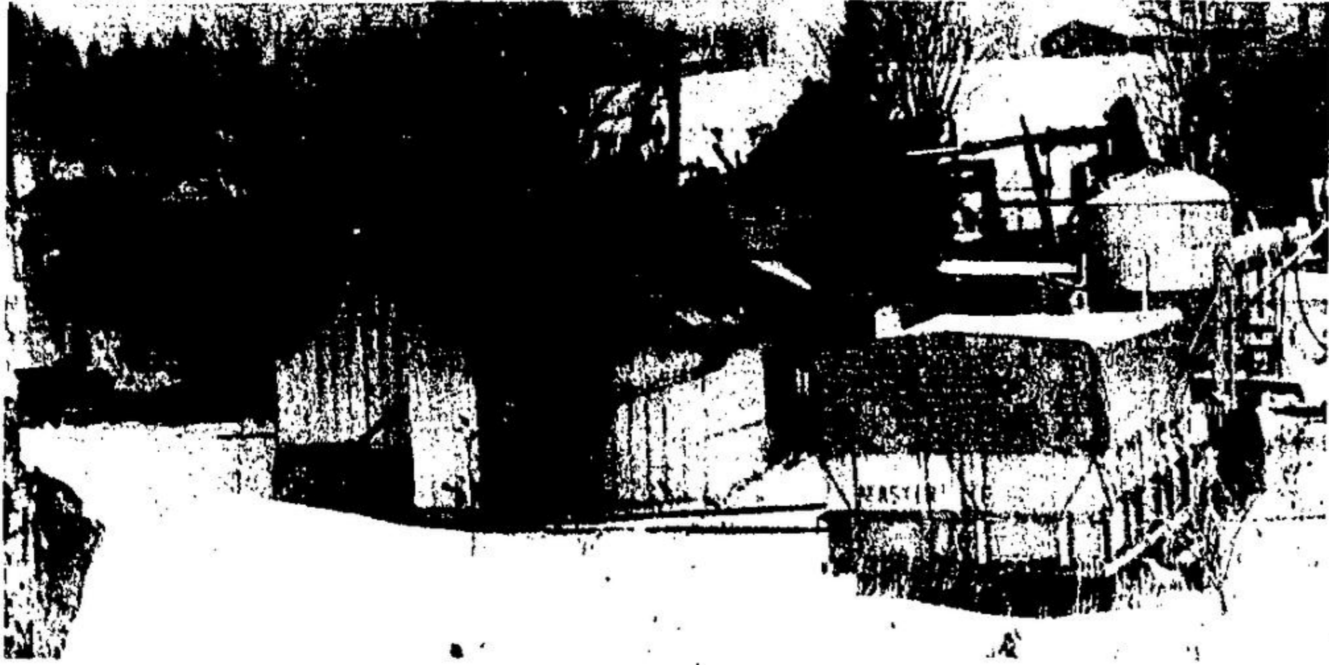
ONLY THE SHELL of the Master Feeds mill at Stewarttown remains standing and hosed down by firefighters after a fierce fire early Tuesday morning. It is the third mill to be burned on the site, long a magnet for farmers in the district. The adjacent store was not touched.—(Staff Photo)
