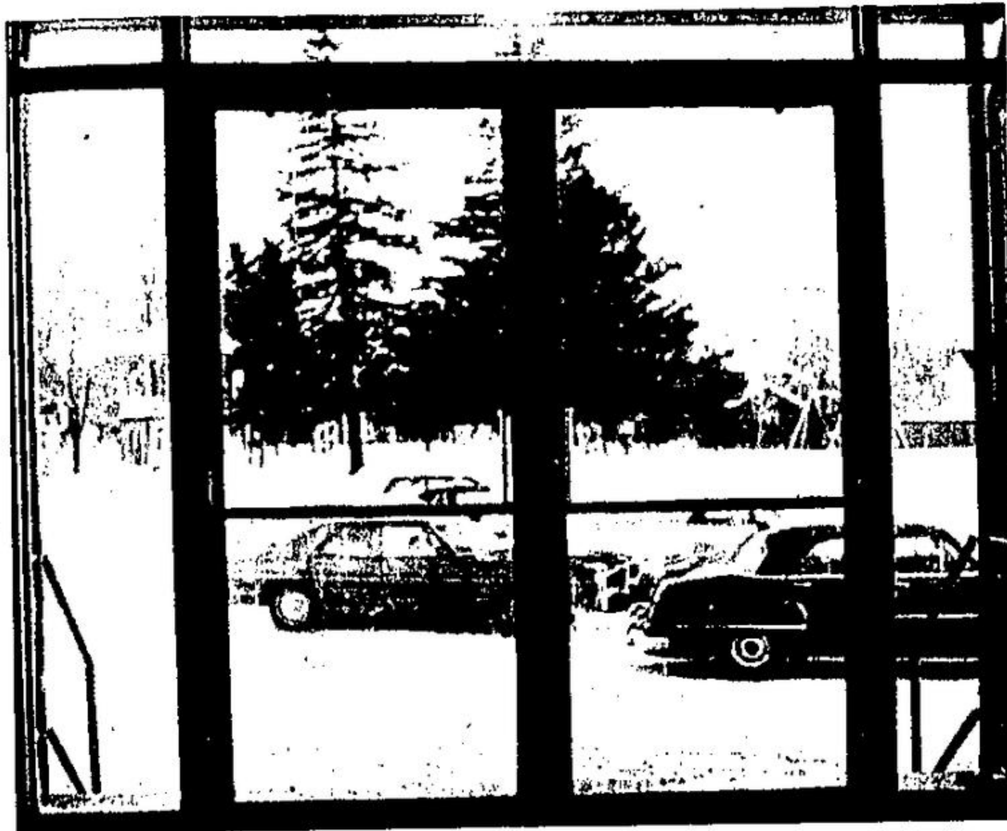
GLASS DOORS have been installed at the giving the building a bright new look.—(Staff entrance to the Acton Community Centre. Photo)
