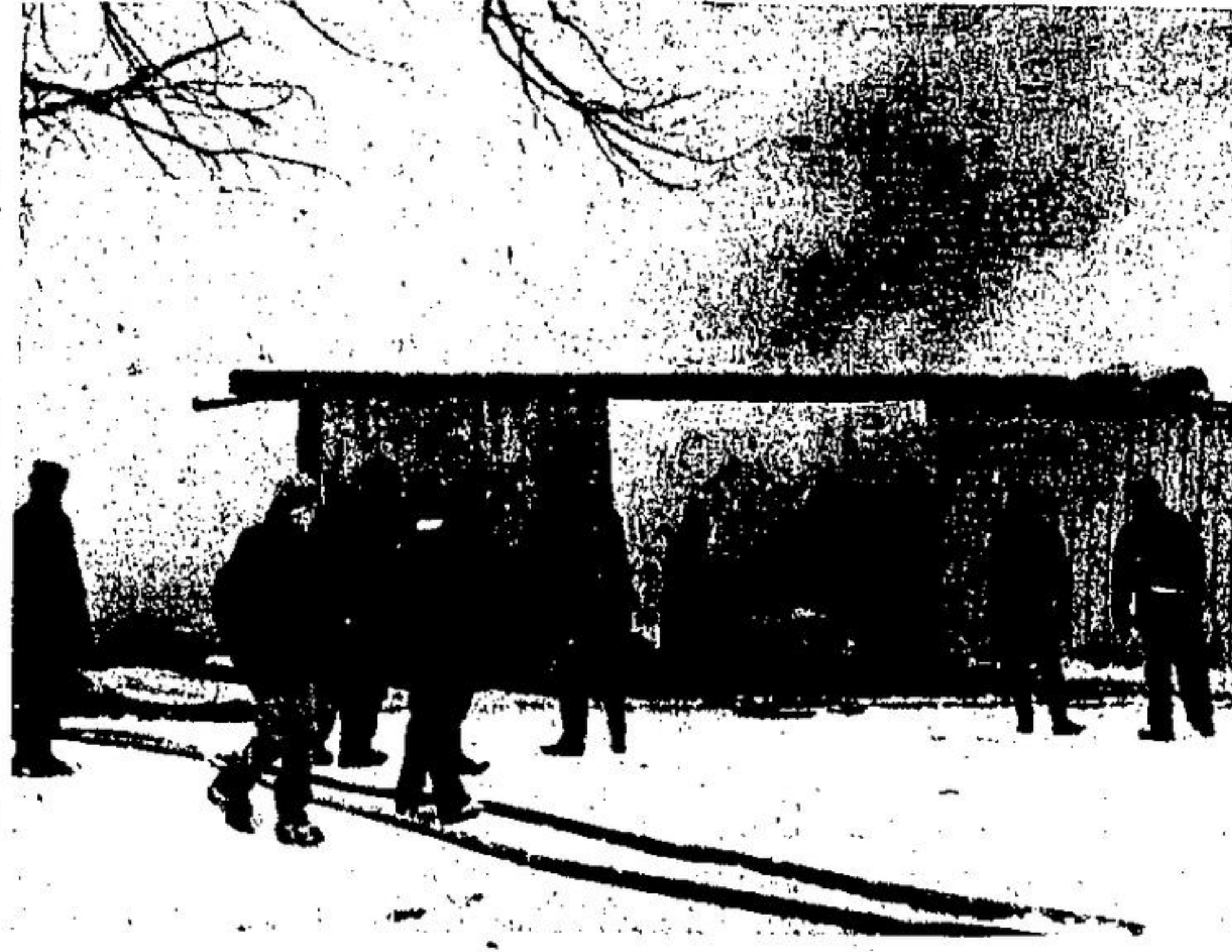
FIRE RAGED THROUGH THE combination workshop and garage of Ron Saunders, R.R. 2, Acton, last Saturday afternoon, completely destroying the building and contents. Mr. Saunders managed to get a car and truck from the building before he was driven away by heat.—(Staff Photo)
