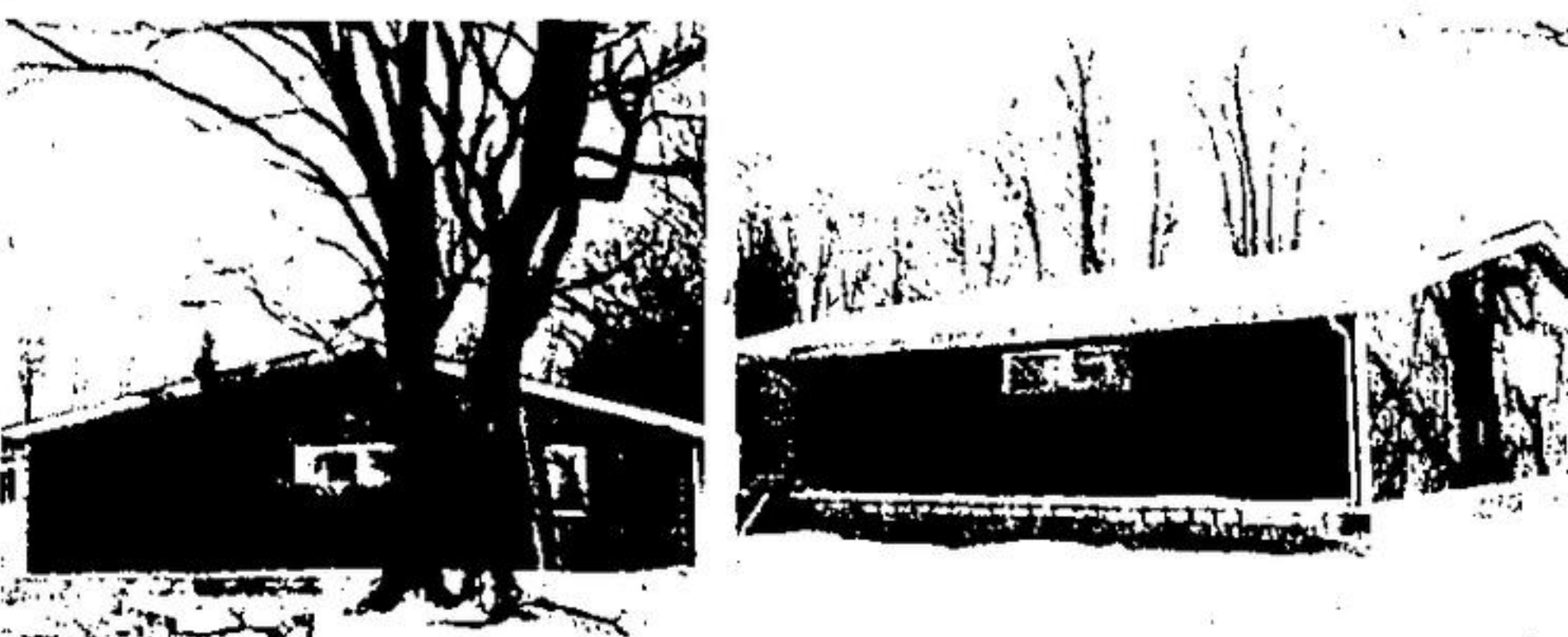
ROCKWOOD'S POST OFFICE in its finishing stages is built of red channel ply-wood. It has a glassed in door area in front, two small windows on one side and two other small ones at the back. At the present time if left as is, it will require considerable indoor lighting installations to allow workable lighting conditions.—(Photo by Lorraine)
