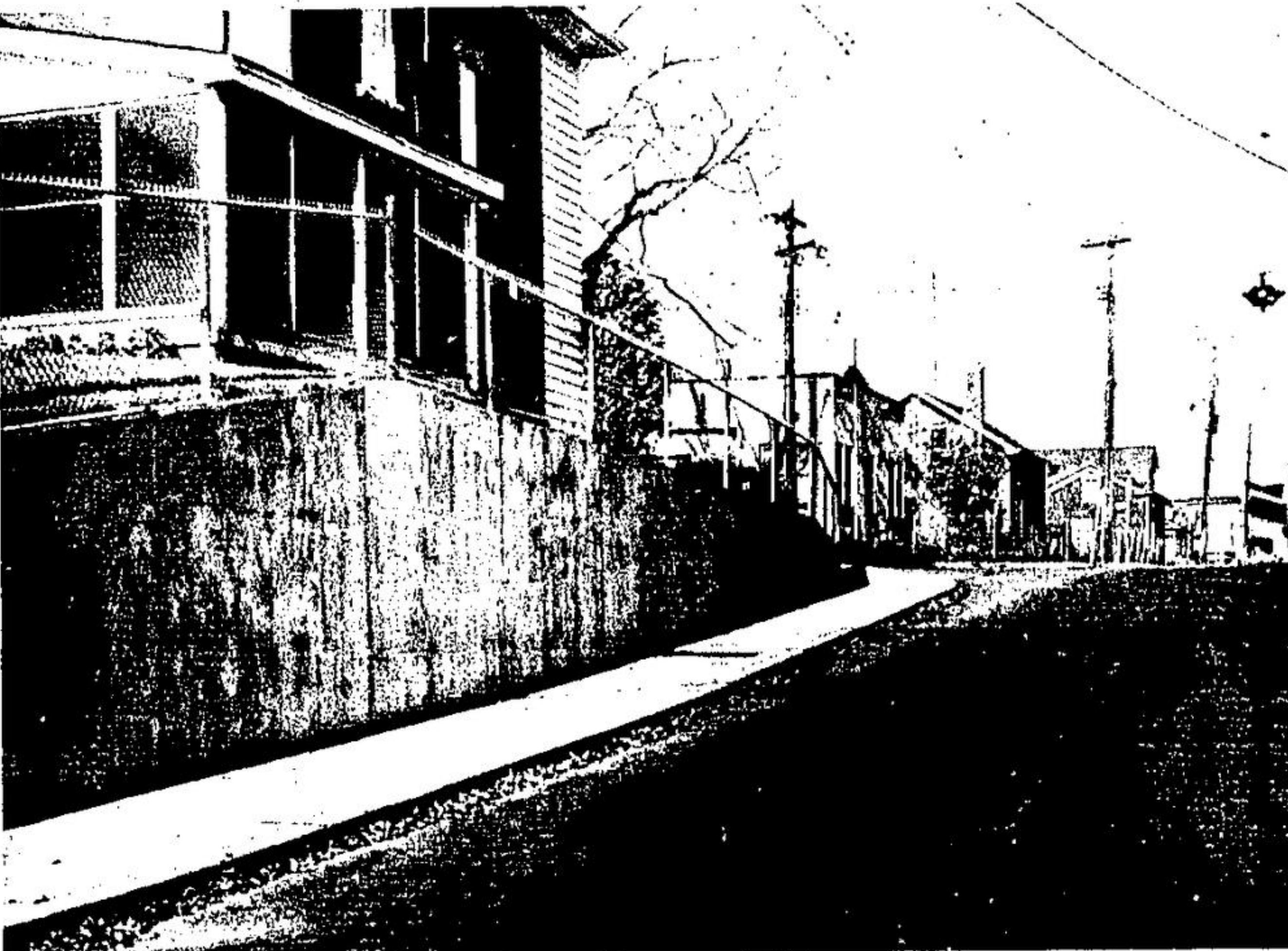
RECENT IMPROVEMENTS at the corner of Mill and Park streets have given the corner a bright new appearance. Cars approaching the intersection on Park Ave. no longer have a blocked view of cars approaching from the right on Mill St. A chain link fence, retaining wall and sidewalk have also helped dress up the corner. —(Staff Photo).
