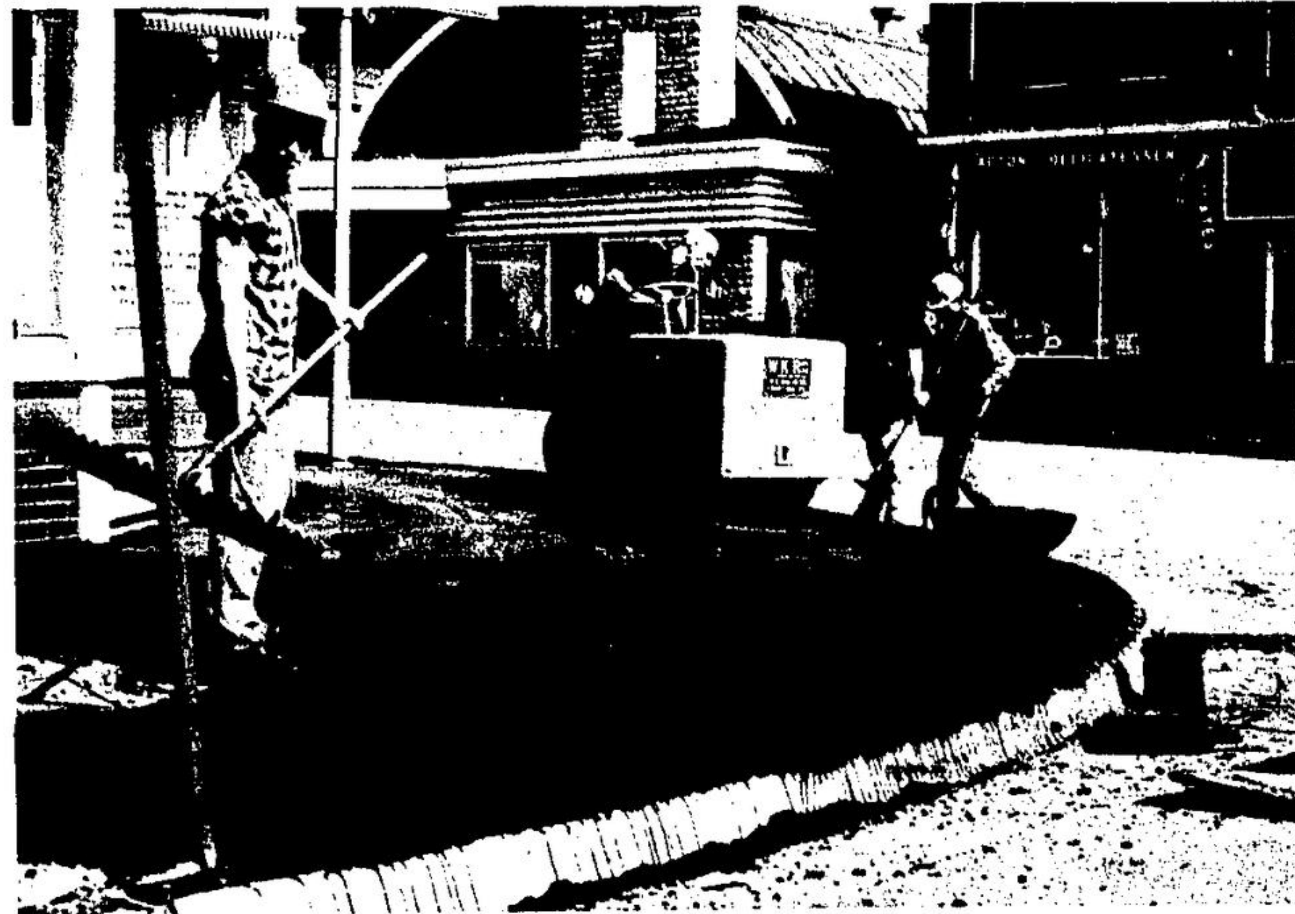
ASPHALT RECAPPING of sidewalks in the downtown area is being done this week by the Milton Paving firm. A two inch compacted surface is being applied.—(Staff Photo)
