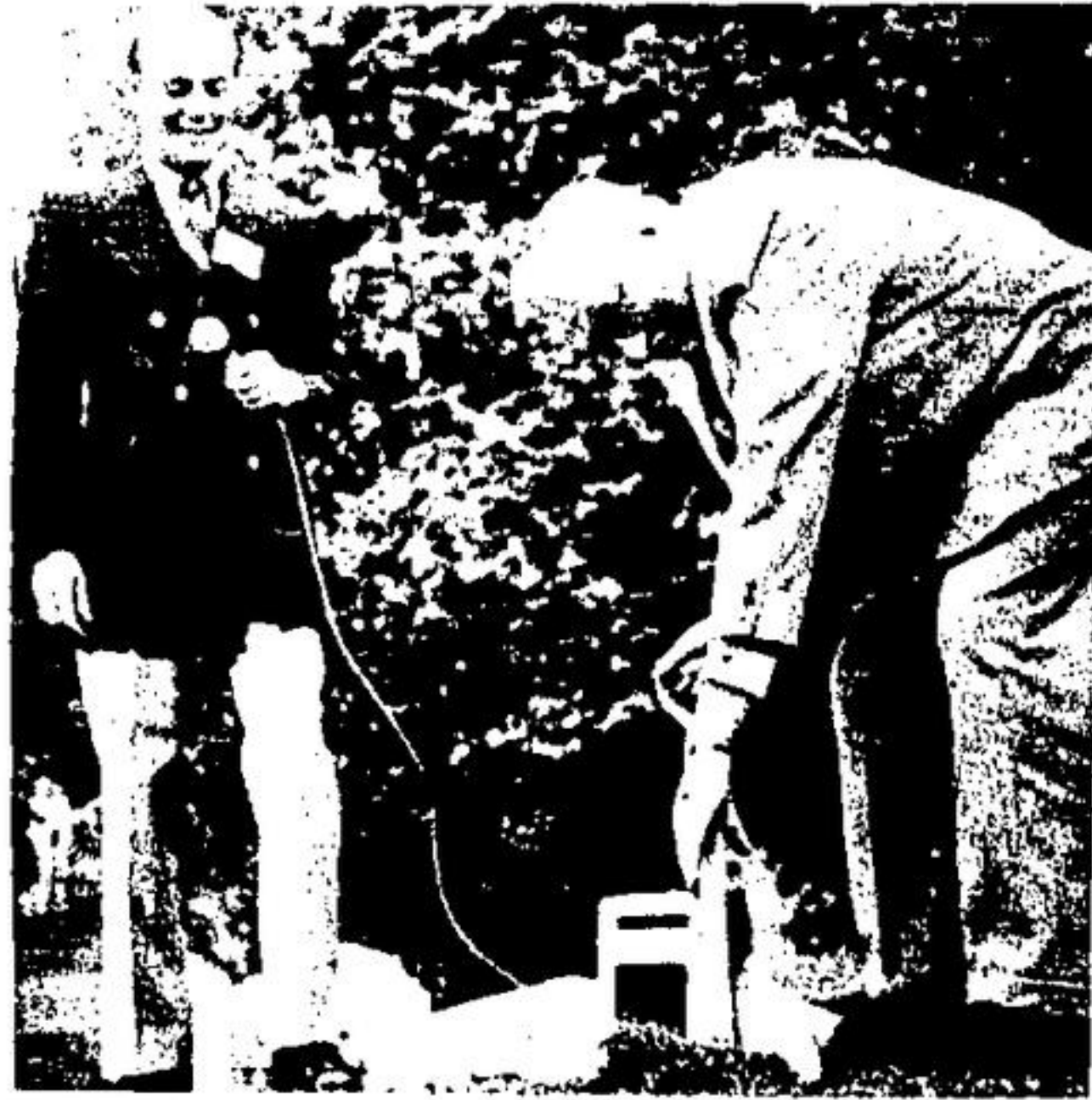
WELLINGTON-DUFFERIN M.P.P. John Root turned the sod to mark the start of construction of nine extra holes at Erin Heights Golf and Country Club recently. Looking on is club pro Bill Richardson. —(Staff Photo)
