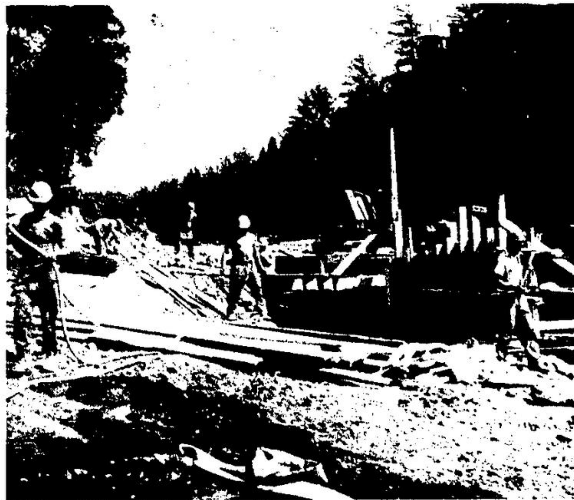
THE FOURTH LINE diversion in Eramosa township is well on its way to fall completion. The bridge semi-structure replaces the old mill building land mark across from Harris lake and the officials of the Phillips Planning
