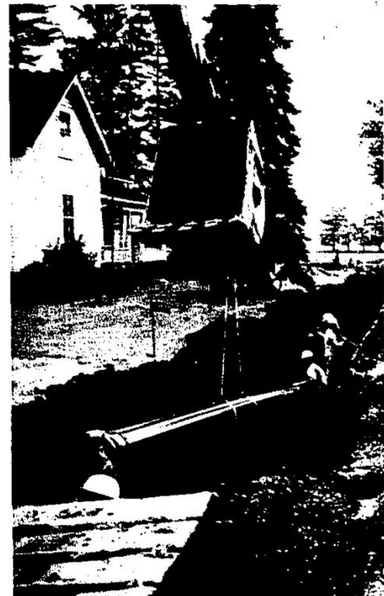
30-FT. LENGTHS OF PIPE are lowered into trench where contractors join them with cast iron flanges. The length of the PCV pipe and its weight ensure fast installation as opposed to short, heavy, competitive types.
