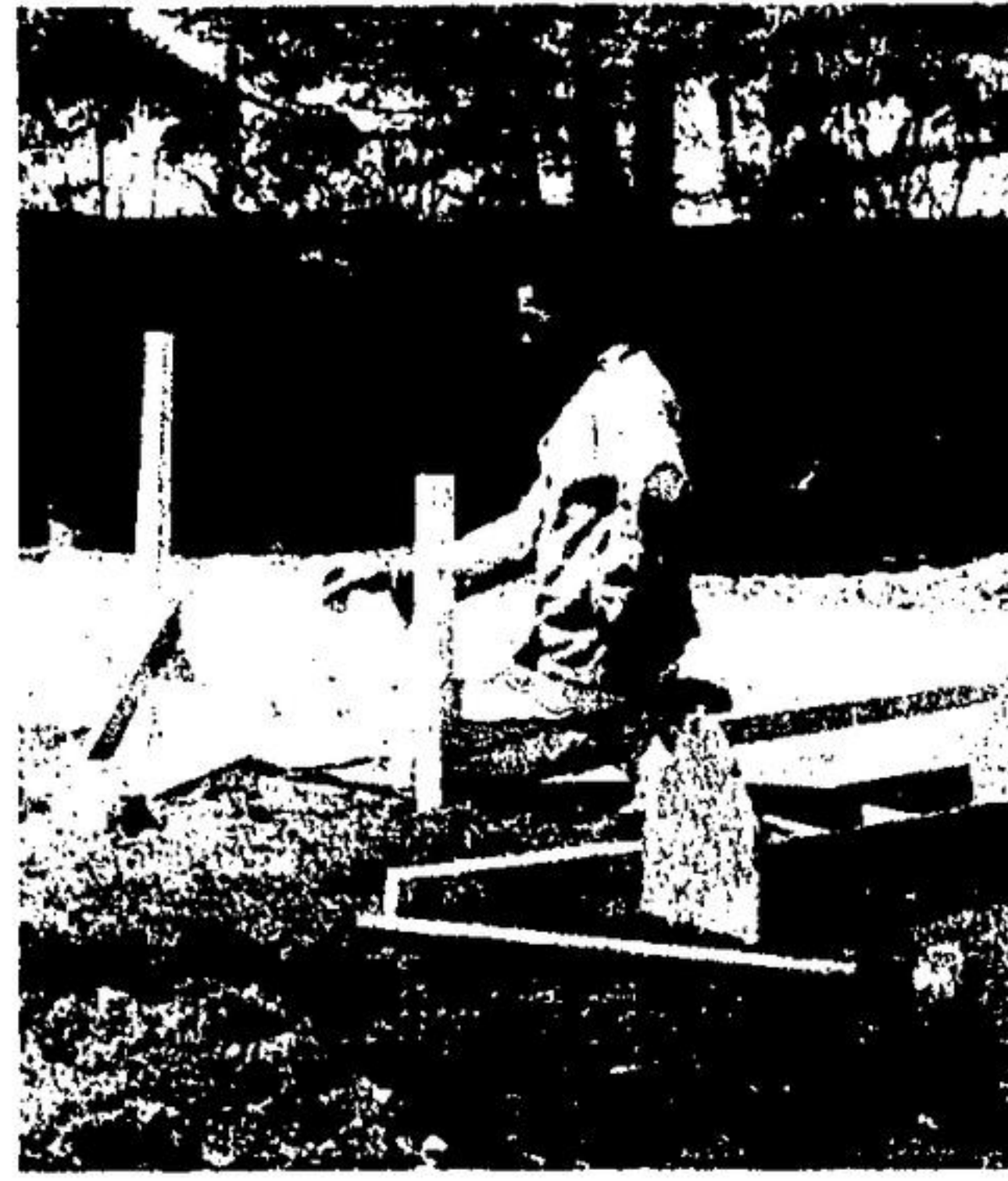
OSCAR CAMPBELL of Ariss takes levels for Lloyd Nellis for the construction of a 110,000 gallon stabilization and mixing plant. —(Staff Photo).
