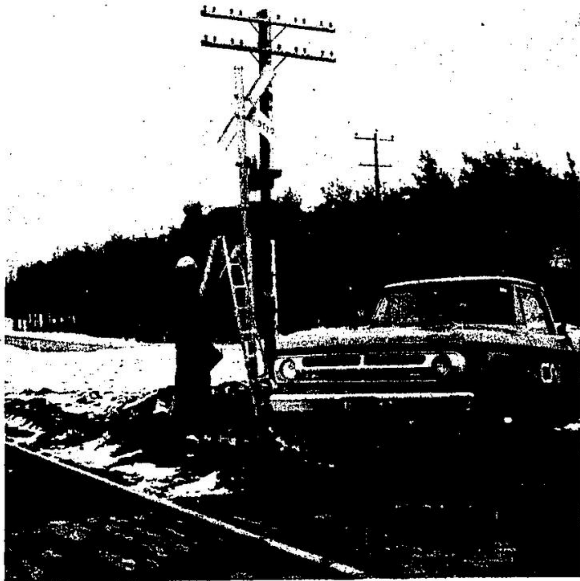
SIGNALS WERE INSTALLED on the First Line Esquesing railway crossing, half a mile west of Acton, by workmen from the CNR. Work started on the installation soon after a car-train accident involving Mrs. Bernice Gibbs, who escaped with minor injuries, although the front end of her car was sliced off completely. The installation had been approved only a few hours earlier by Esquesing Council. —(Staff Photo)
