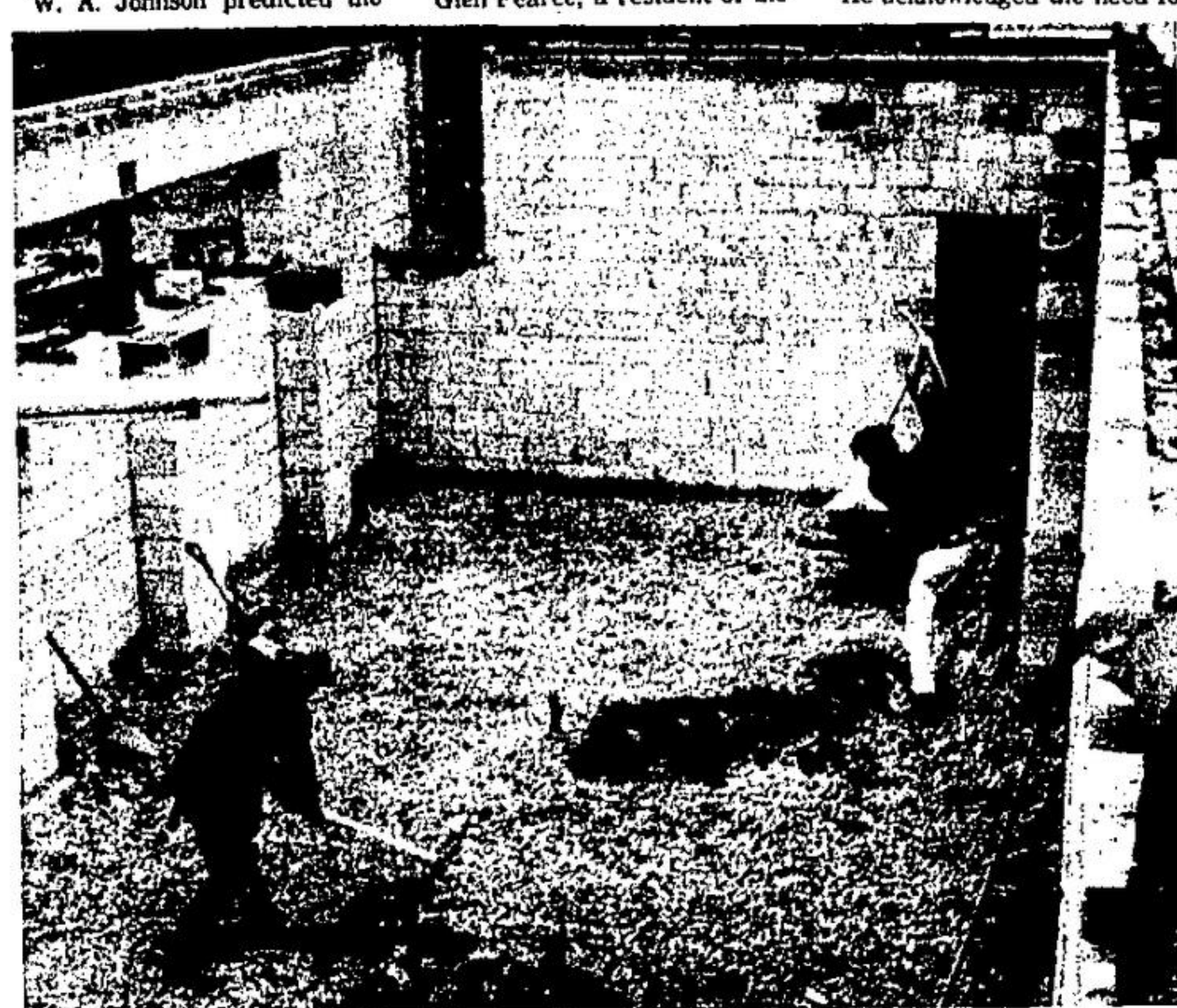
THE BASEMENT of the new addition to ARC Workshop, Hornby, is still under construction. Due to delays the building scheduled to be completed by November will not be ready until the end of December, reported supervisor Mrs. W. Isham. Workmen are preparing to lay the cement floor. To raise money for the new addition an auction sale has been planned
