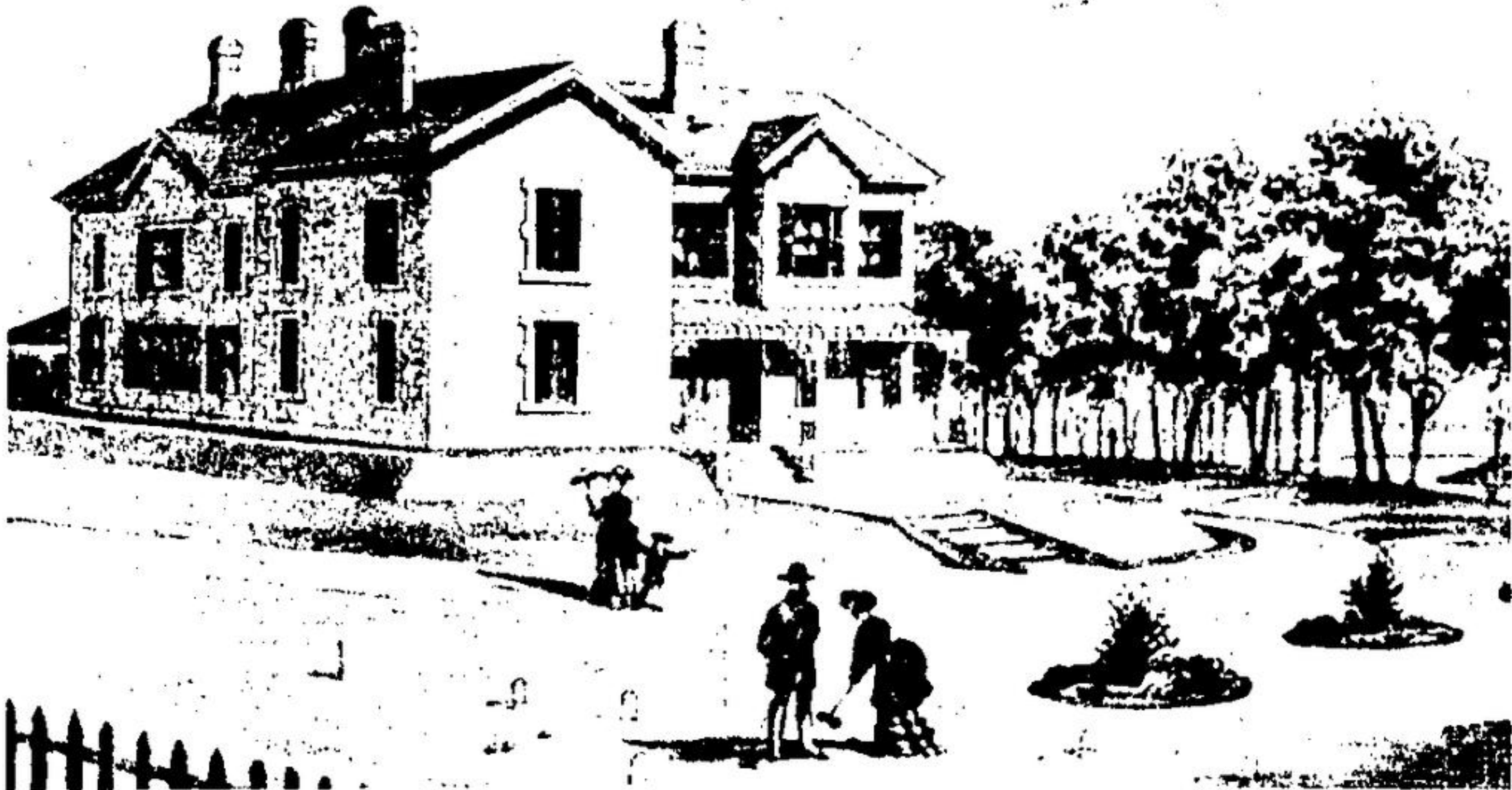
THE FORMER ACTON HIGH school and now part of the Robert Little school, the former Sidney Smith residence still preserves much of its character. Art teacher Bob Bateman urged students at the high school
