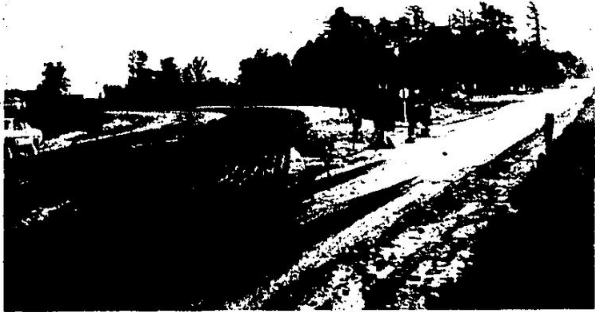
BESIDES MAKING a wider curve, reconstruction of Highway 7 will allow for a one way entrance on to Trafalgar Road South and a two lane entrance
