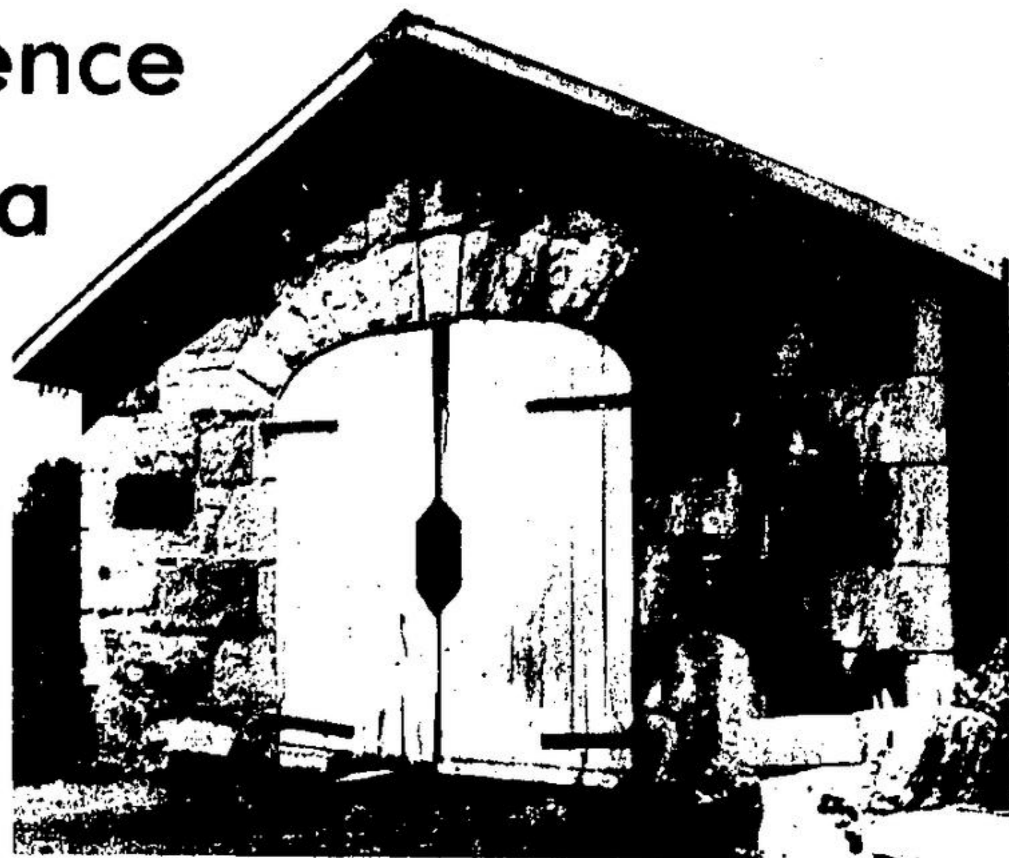
A GREAT DEAL of effort and know how went into the placing of hand-cut stones in buildings such as this garage, on the farm of Wallace Lasby. The stone
