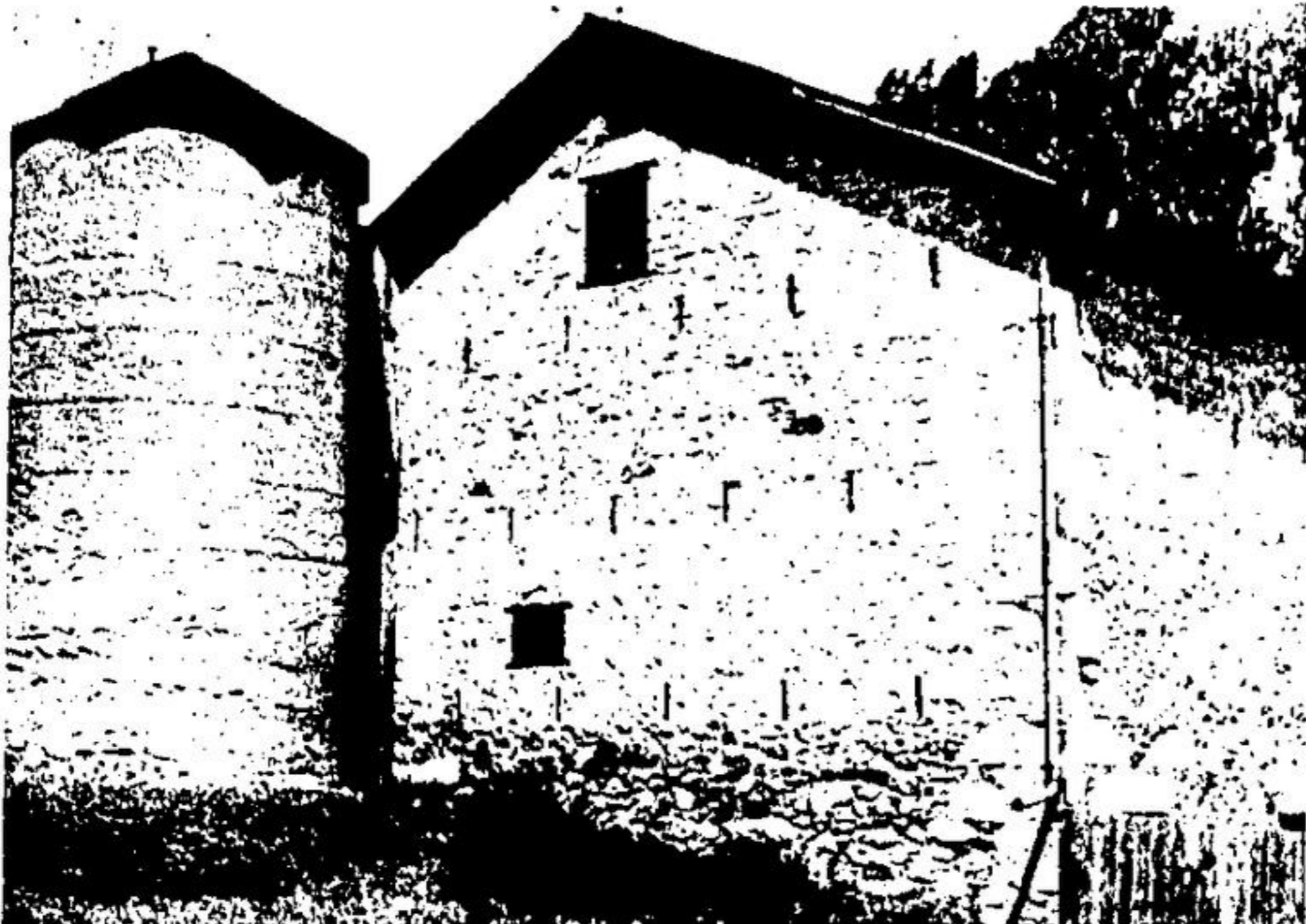
A SILO 20 feet high, which extends 15 feet below the ground as well, is attached to the stone barn on the farm of Robert Croft on the Guelph Line. The
