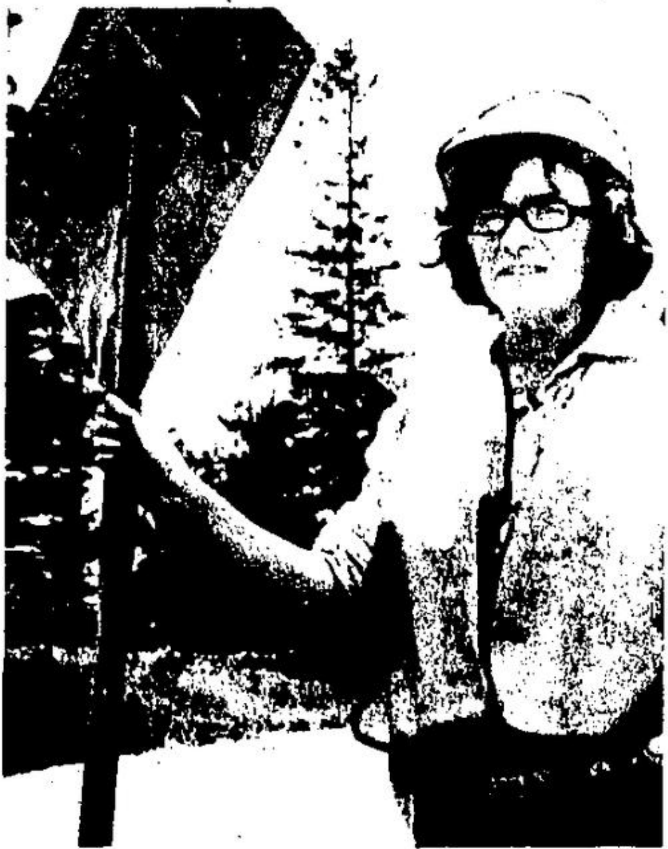
BARBARA LAWLER of Maxwell Ontario, near Flesherton is one of three high school girls being employed as flag girls on the reconstruction of Highway 7, east of Acton. The girls work a regular eight hour day for Harry Hamilton Construction Ltd. of Nottawa Ontario.—(Staff Photo)
