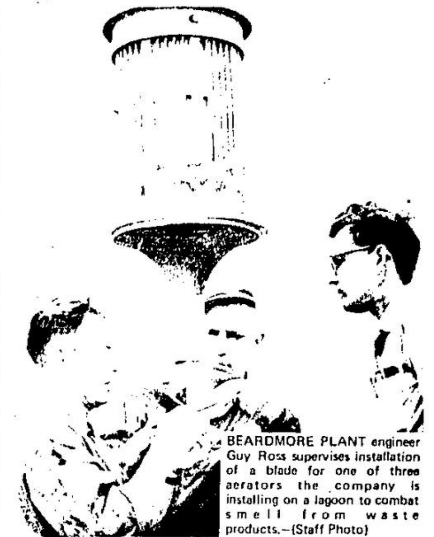
BEARDMORE PLANT engineer Guy Ross supervises installation of a blade for one of three aerators on a lagoon to combat smell from waste products.—(Staff Photo)
