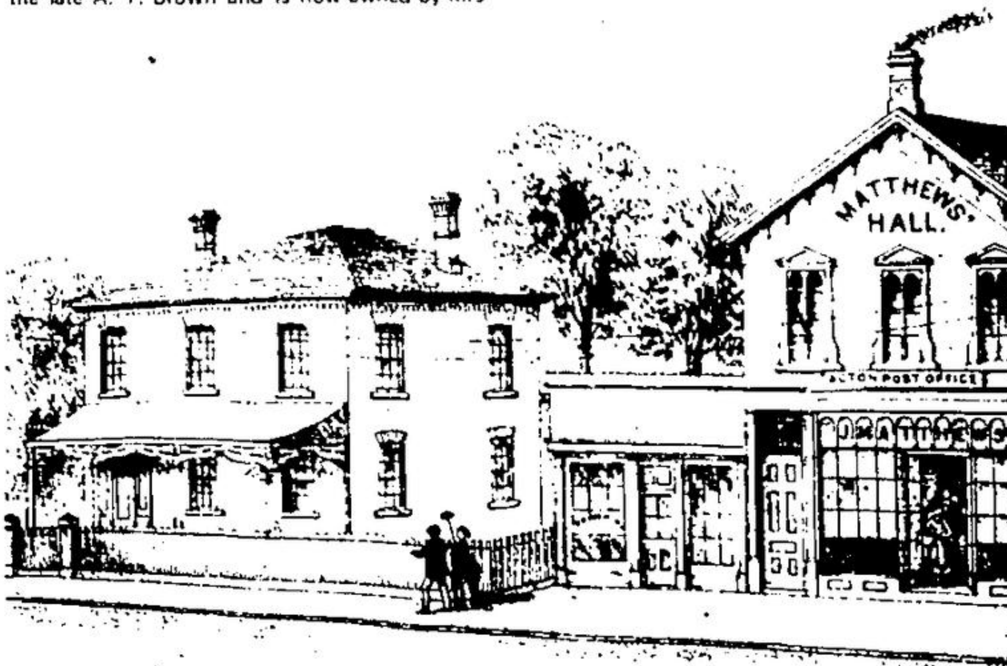
STORE & RESIDENCE OF J. MATTHEWS ESQ. ACTON WEST.
