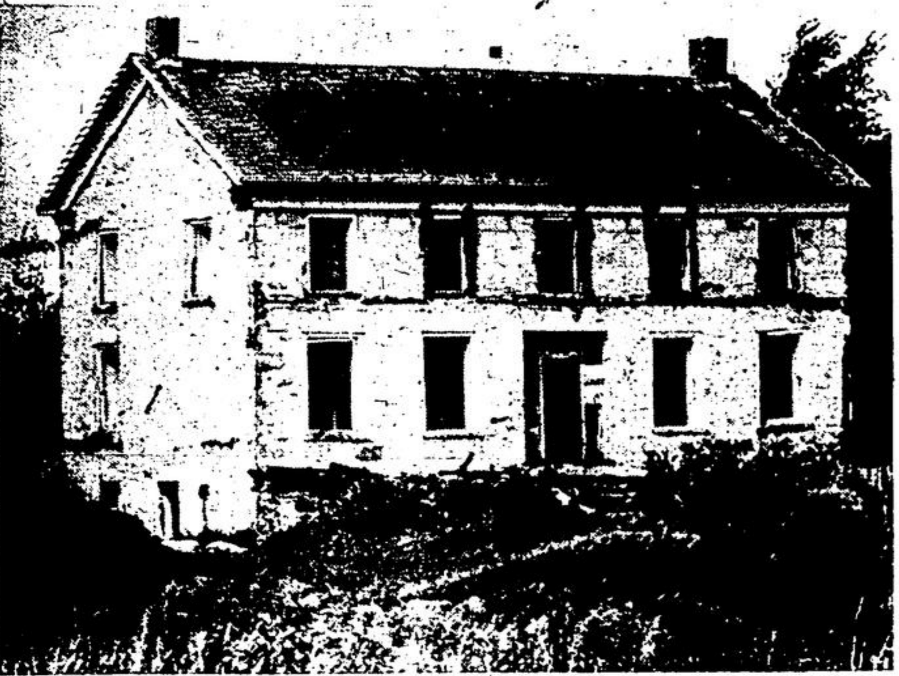
Now empty and gutted, the house has lost its stately appearance. It has been stripped of its valuables and is now nothing more than an empty shell.
