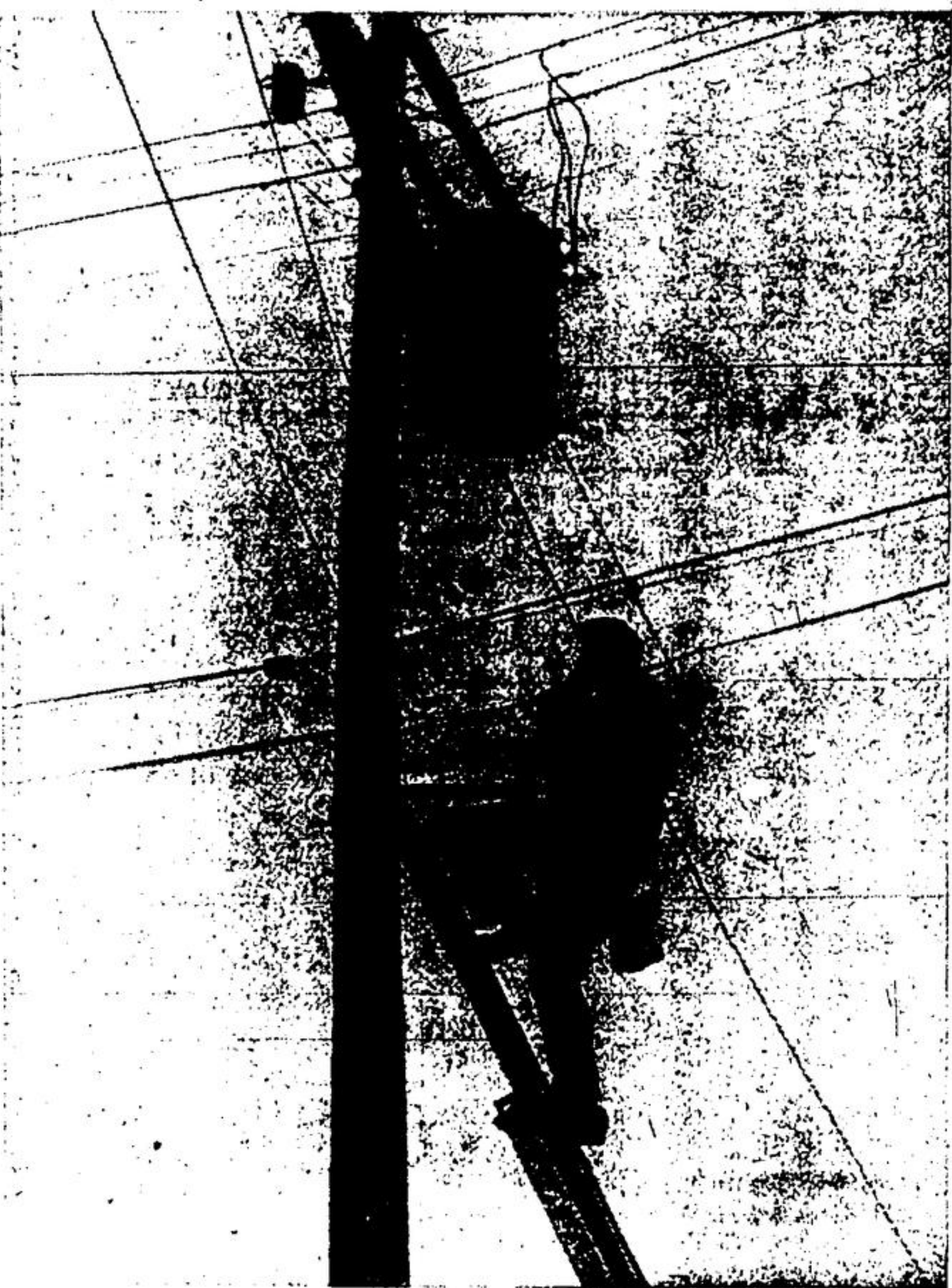
CLAMPING A PRESSURE TAP to one of the distribution cables John Ollivier of Georgetown Cable TV completes the hooking up of a subscriber's set. Most of the streets between the company's tower atop Norval hill at the eastern town limits and Maple Avenue now have the distribution cables on their poles. Antennae will start disappearing from local rooftops as the service reaches more subscribers.
