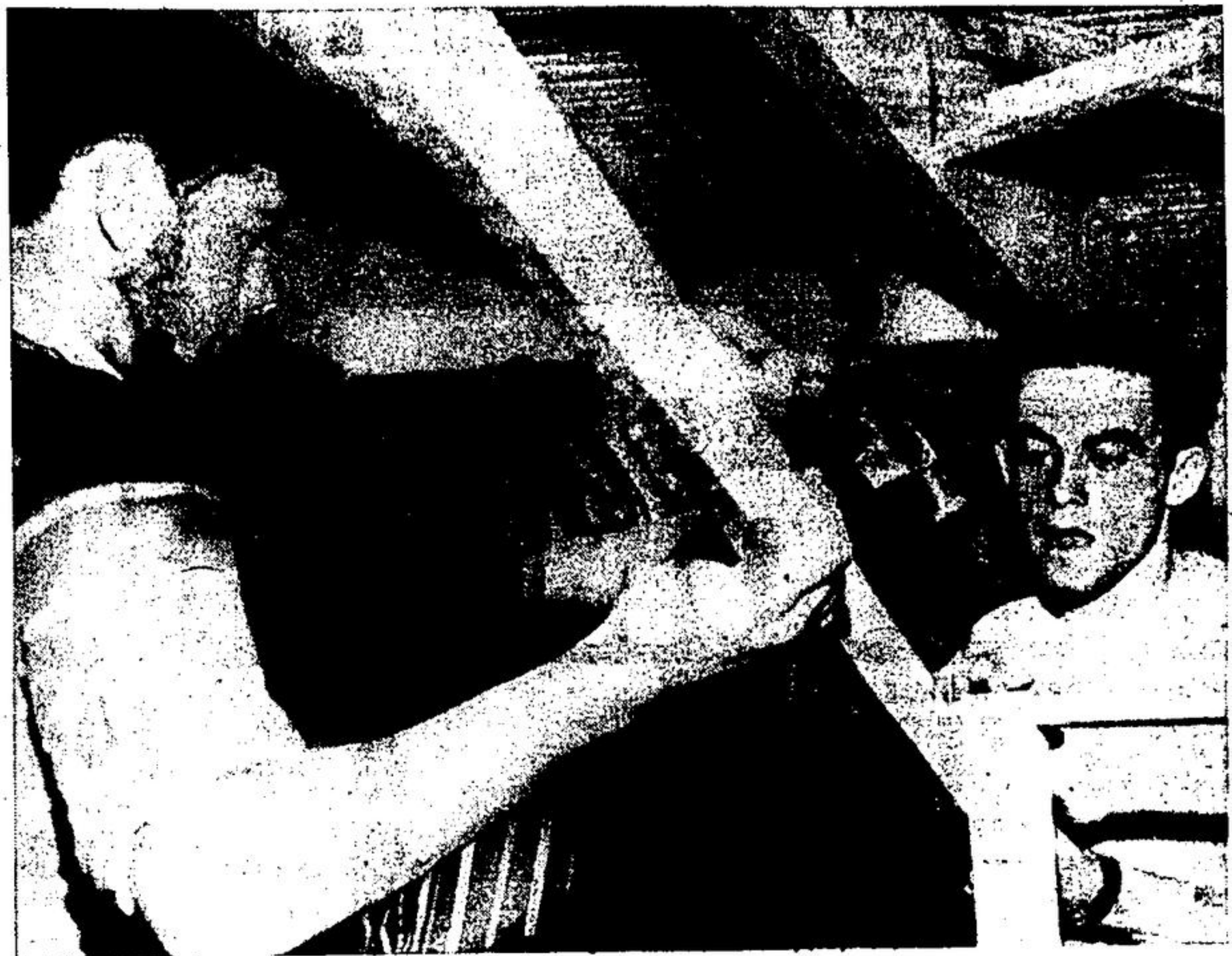
GARY GLAUDE AND JIM EGERTON hold a cross brace for Finn Poultrop as Youth-in members go about converting boiler room to coffee house.
