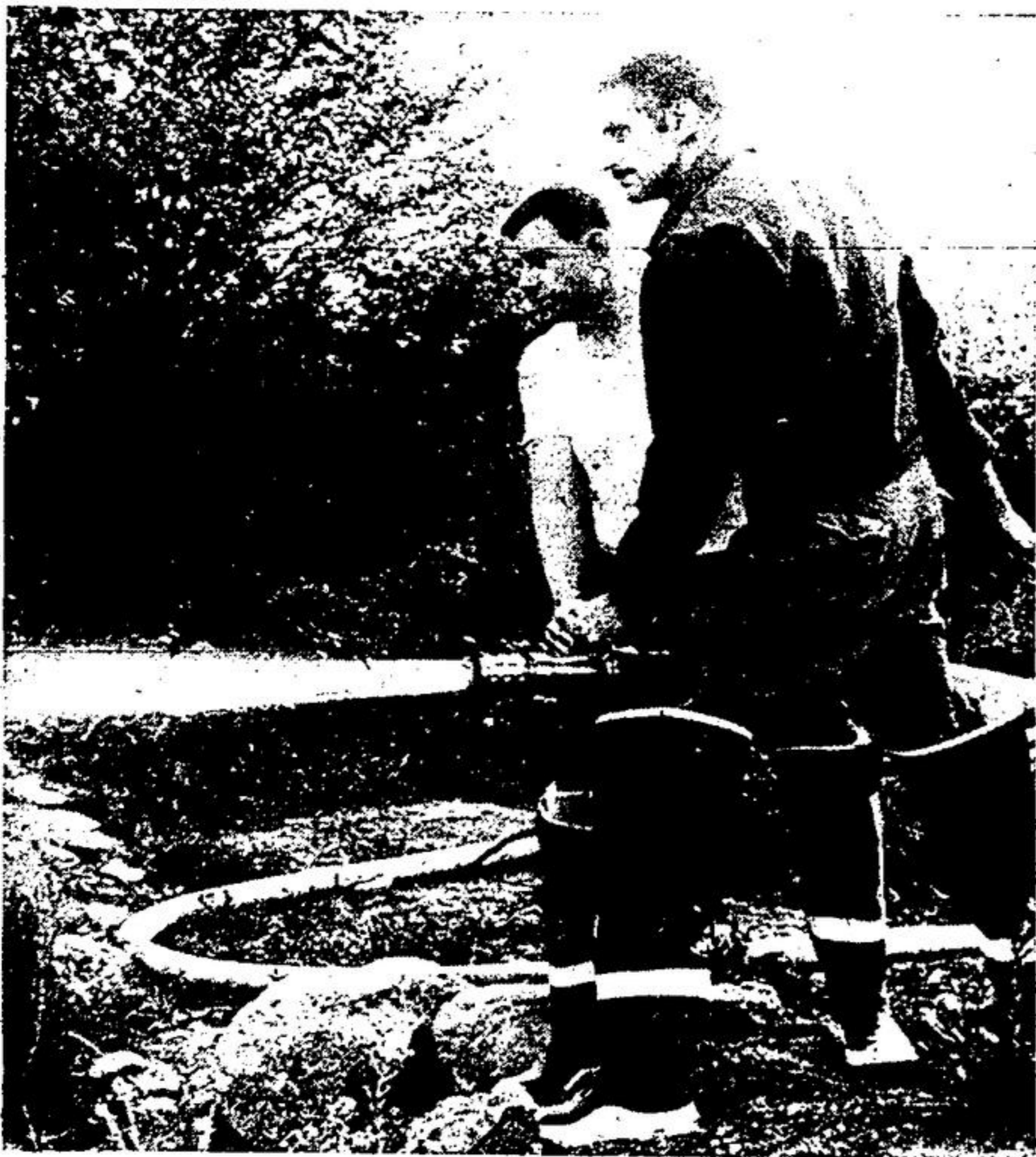
Bud Hyde and Tom Massena, added to fire department
