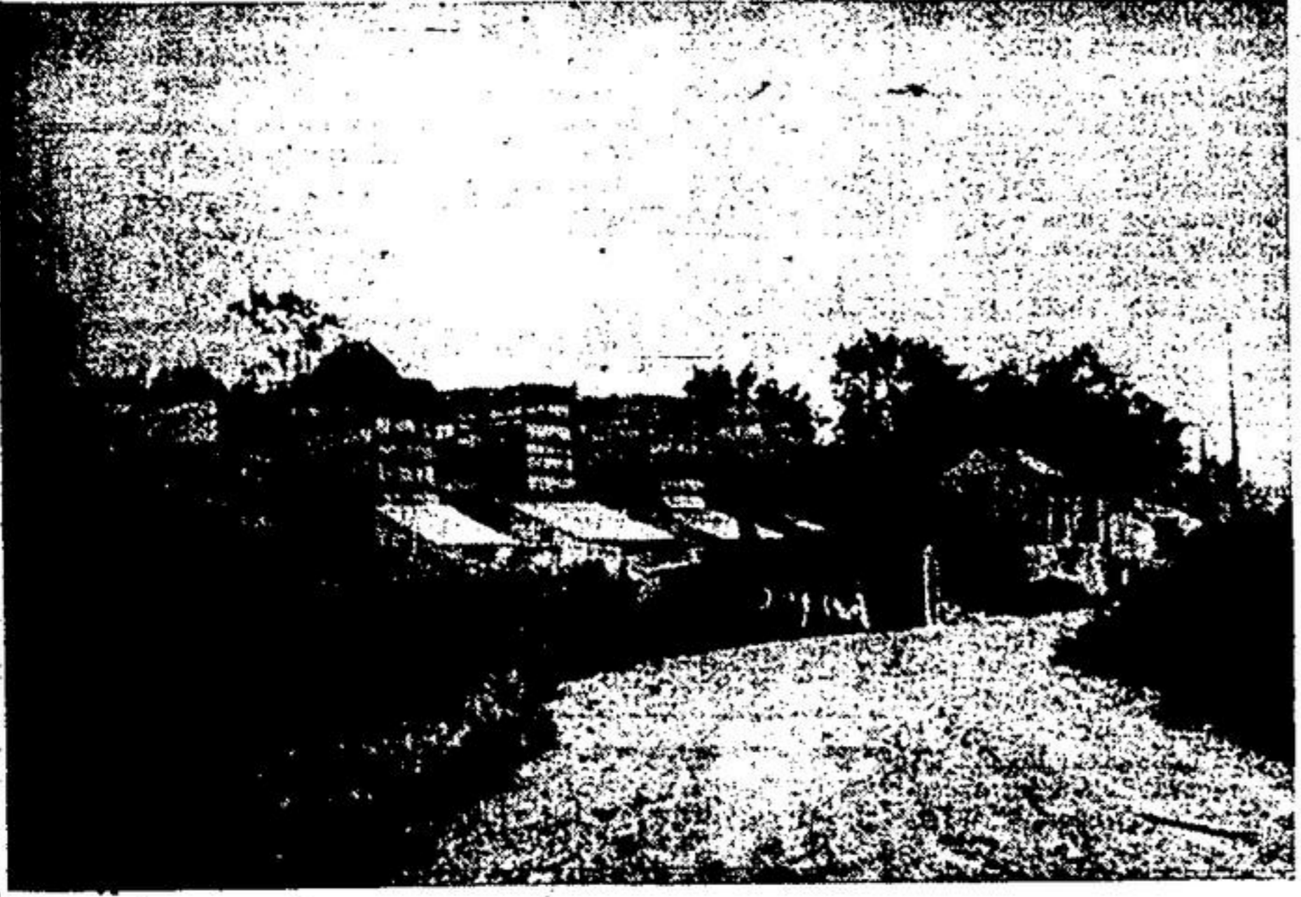
LOOKING LIKE SEVERAL oddly-constructed beehives, these kilns provided employment for more than 100 men when this picture was taken about 1900. Limestone was blasted from the nearby quarry and drawn to the kilns by horse and wagon. Here it was fired into lime for uses in early Ontario.
